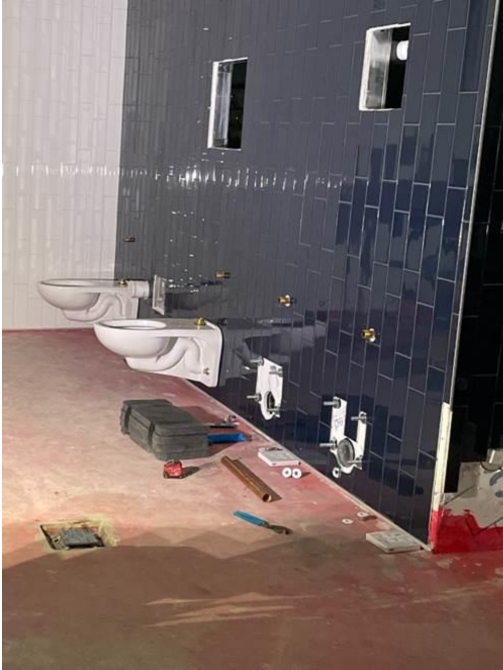
Toilet installation in the main locker rooms
