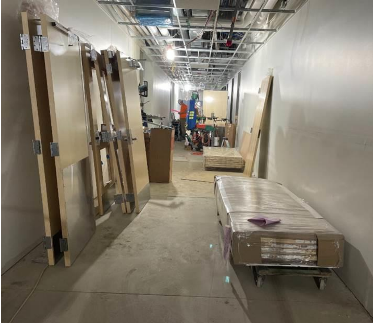
Door installation on the Academic Wing's first floor
