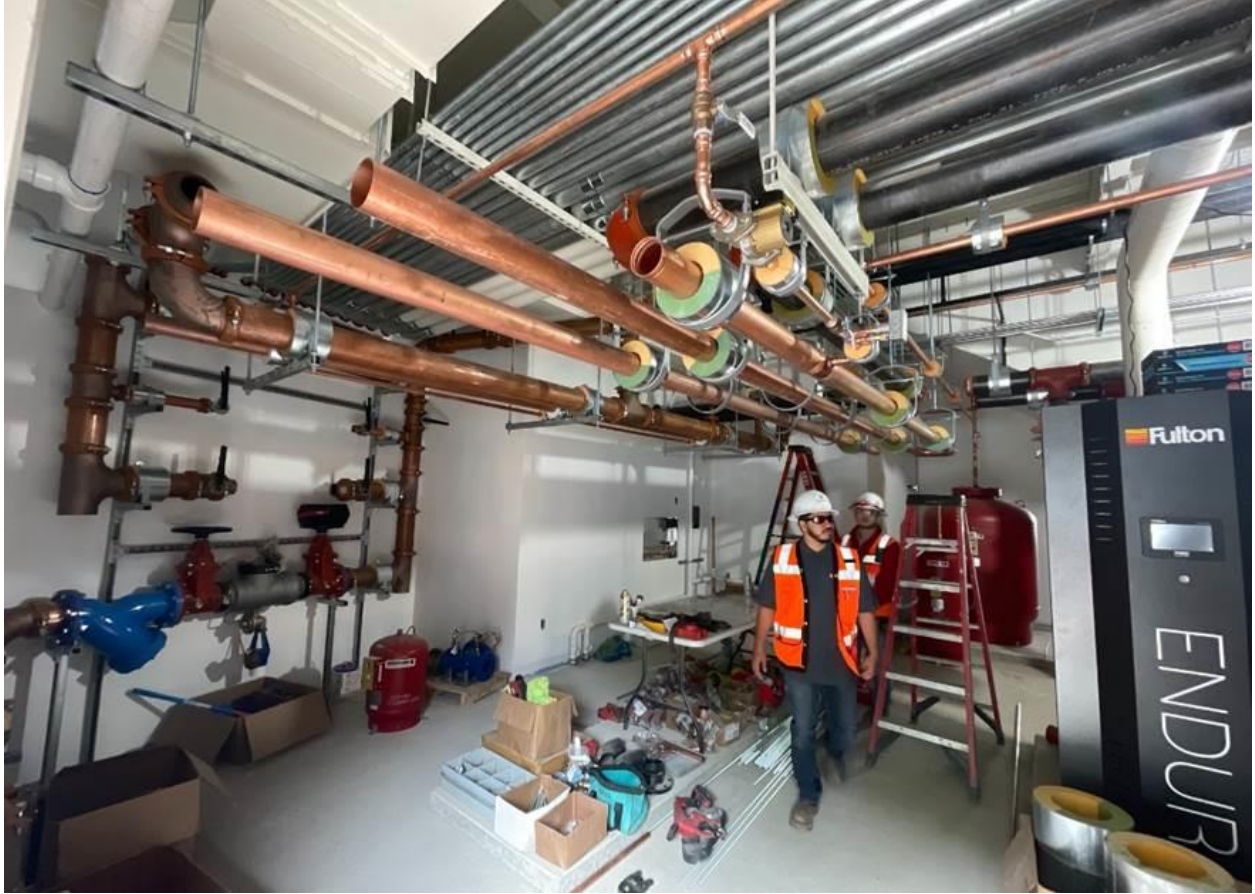
Final connections being made to the buildings' primary water lines
