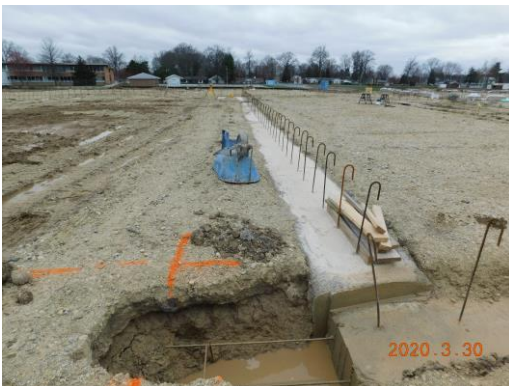
Unit B footing and rebar
