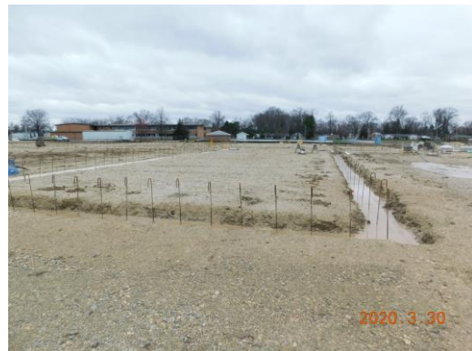
Unit B footings and rebar
