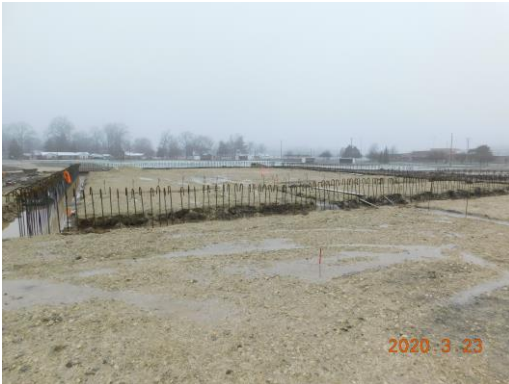
Unit a gym foundations and rebar
