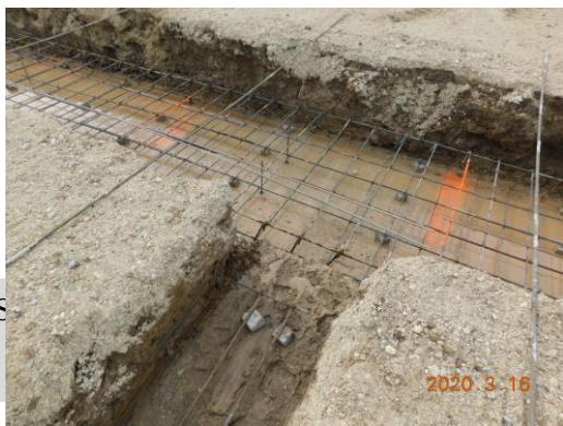
Rebar placement for Gym footings
