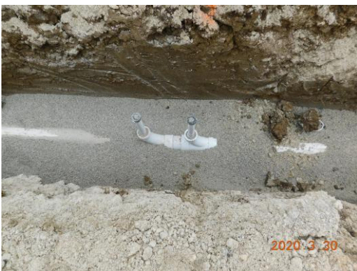
Up close view of underground plumbing install
