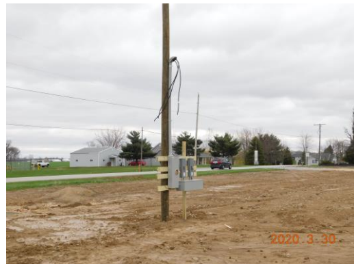
Temporary electric meter install
