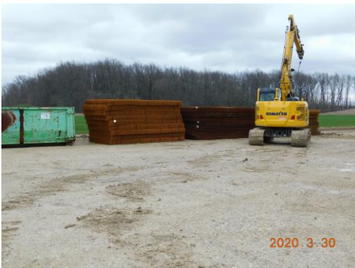
Wire Mesh stored on site for concrete pours
