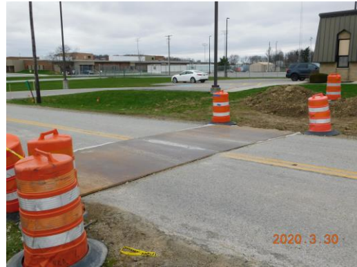
Underground utility tie in across the road from the Admin office to the site
