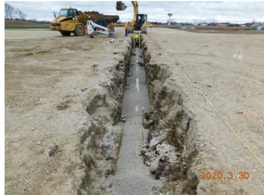
Underground plumbing being installed
