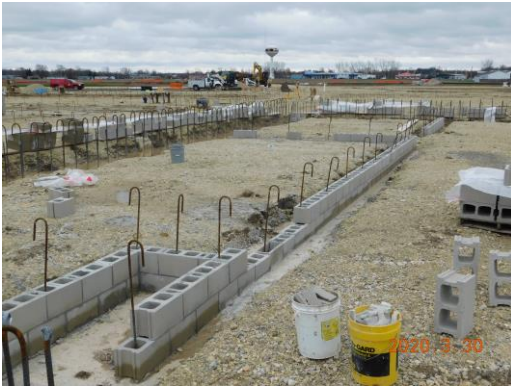
Masonry foundations in Unit A
