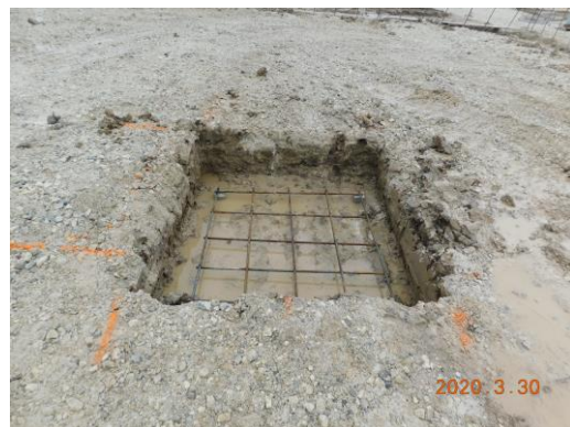
Column pad prep for Unit B with rebar installed
