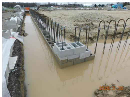
Unit A gym corner masonry foundations
