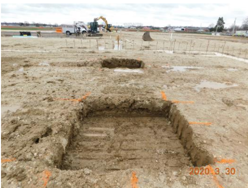
Column pads prepped for rebar and concrete for Unit B
