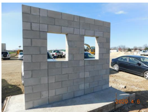
Masonry mockup installed for CMU review
