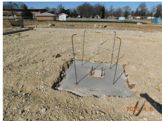
Column footings complete in the media center in Unit B
