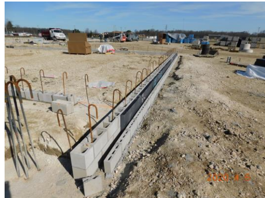
CMU foundation wall with insulation started in Unit B student dining, kitchen area
