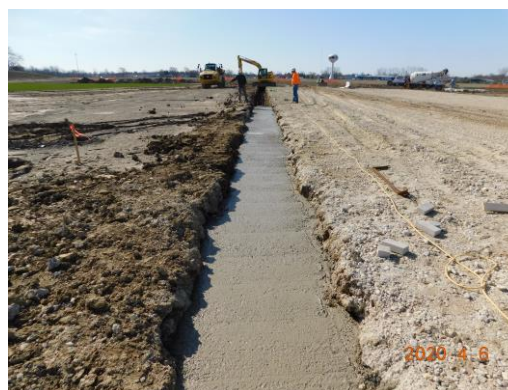
Footings being poured along the Unit E classroom wing
