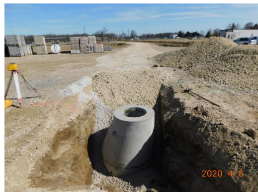
Sanitary man hole installation along the northwest side of the building area
