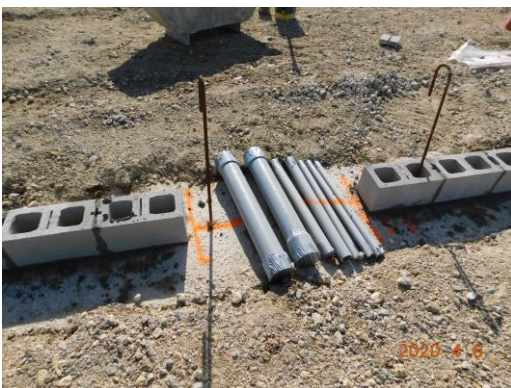
Sleeves for through wall penetrations being laid out and prepped for walls
