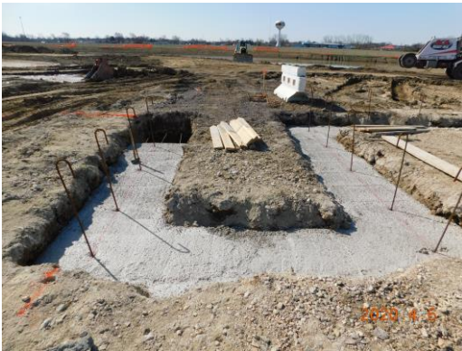
Footing installed for the far south doorway in Unit E classroom wing
