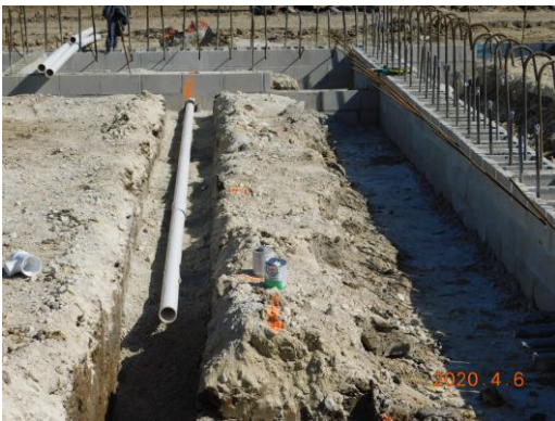
Underground plumbing started for restrooms off the gym in Unit A
