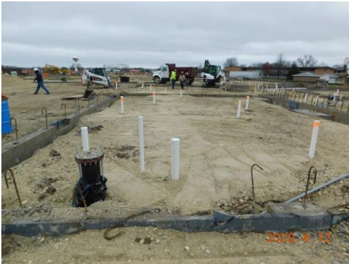
Underground plumbing stub ups in Unit A
