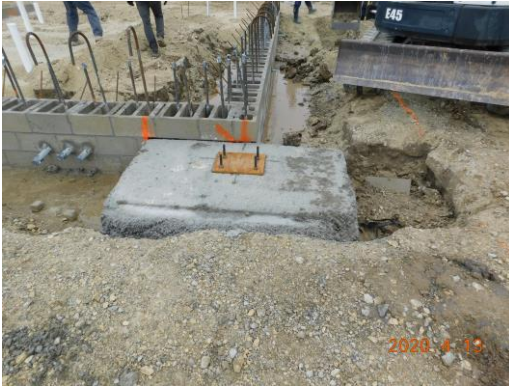
Column Pad outside of Unit A area
