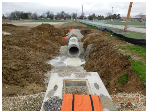
Storm installation along the North side of the property
