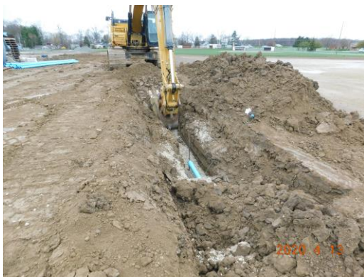
Water line installation North of the new building
