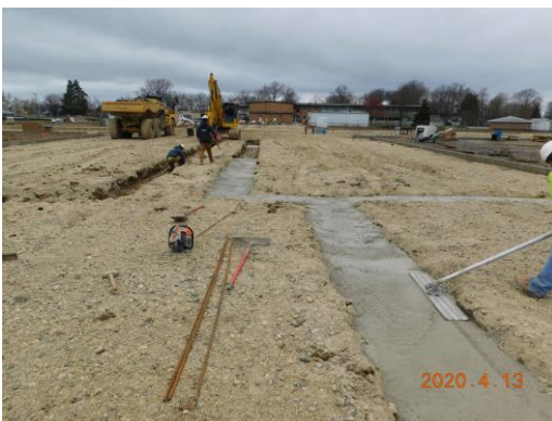
Interior footings poured in Unit C
