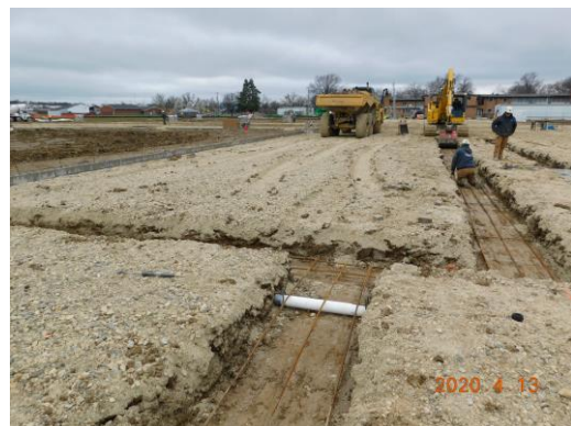
Interior footings being prepped for concrete
