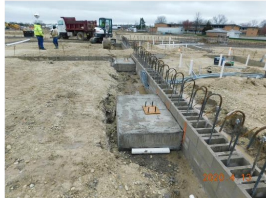
More column pads outside Unit A area
