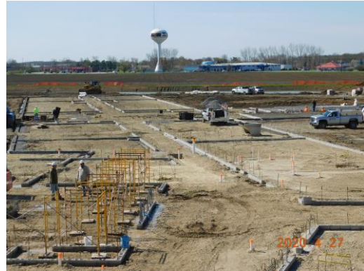
View from the south wall of the gym looking towards the south
