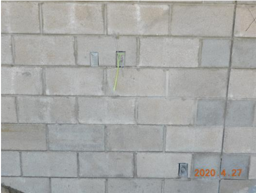
In wall electrical roughs on the south wall of the gym
