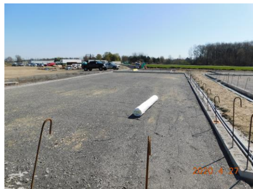
Stone pad prepped and ready for vapor barrier prior to wire mesh install and concrete pour
