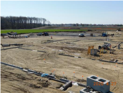
View from the south wall of the gym looking at the cafeteria, stage, kitchen areas
