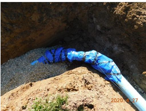
Underground water line installation on the southwest side of the property
