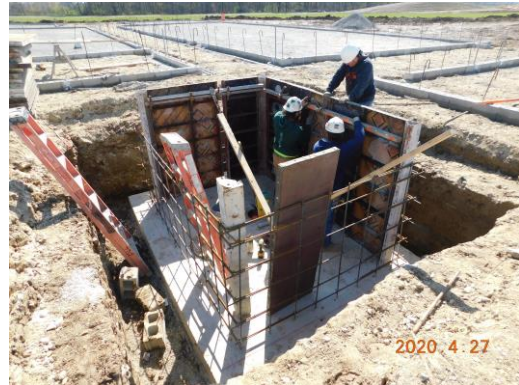
Elevator Pit walls being formed and prepped for concrete
