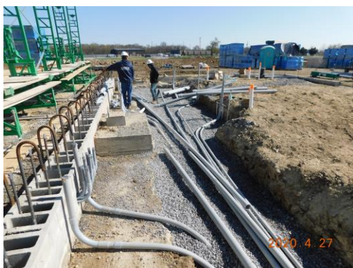
Underground electric being installed to the main electric room
