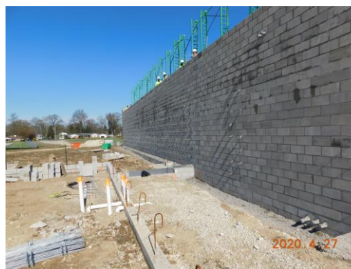
South wall of the gym being erected
