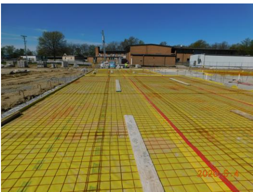
Floor prep taking place in Unit C classroom wing
