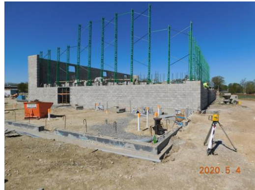
View of gym walls from the northeast side of gym
