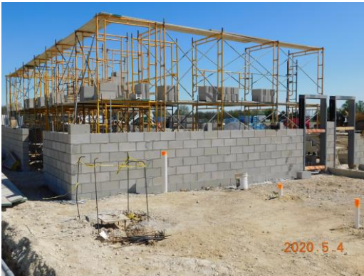
Unit B masonry by the kitchen going up, and doorframes set
