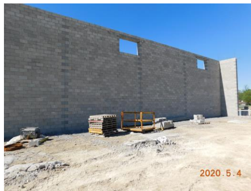
South gym wall taken to bearing height
