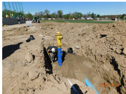
Fire Hydrant installed along the North side of the gym
