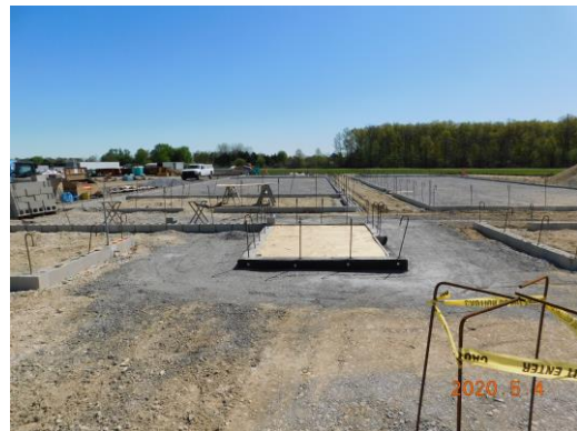
Elevator pit poured and covered to protect it
