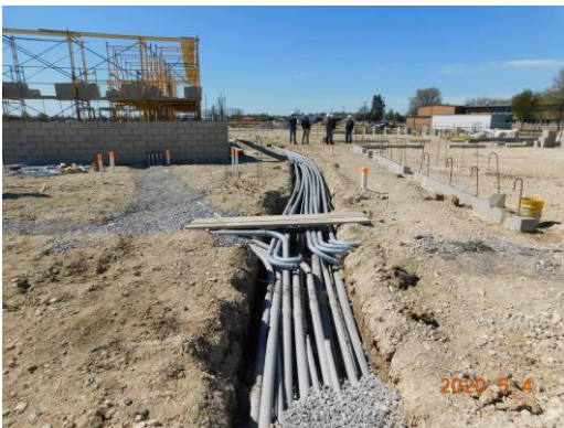
Underground electric duct bank being run down the main corridor from Unit A to B
