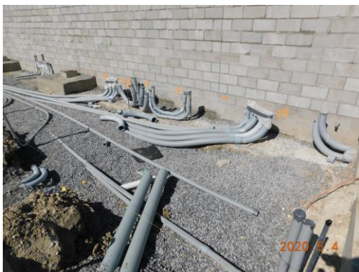
Underground electric being installed to the main electric room to switchgear
