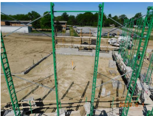
View of the administrative area being prepped for CMU installation
