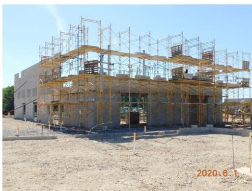
CMU installation around the student dining
