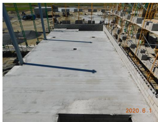
Precast set above the student dining area (unit b)
