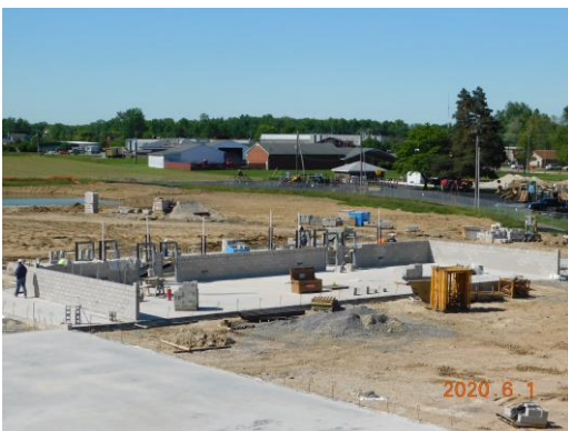
Unit C classroom walls being installed
