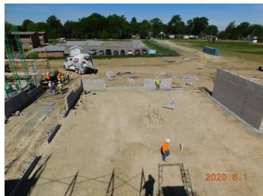
Walls for the media center area being installed
