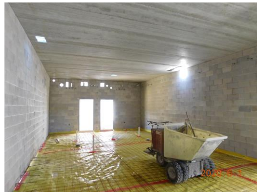
Floor prep under Unit A mezzanine
