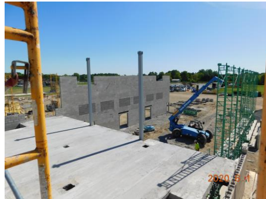
View of the student dining area from atop the precast
