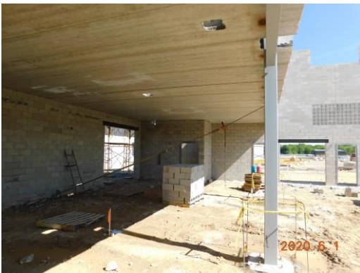
View under the precast of the student dining area
