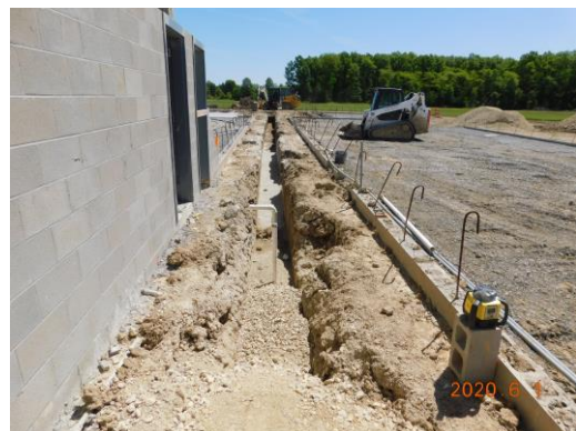
Underground sanitary being installed in Unit D
