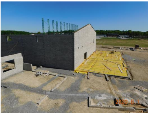
Concrete floor prep and gym walls in unit A
