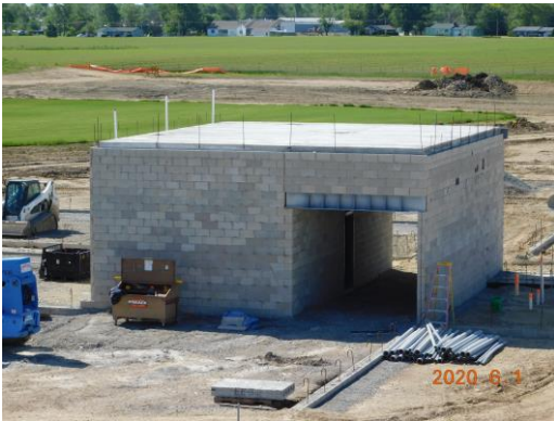
Unit D precast set
