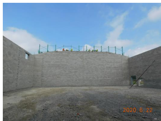
West end of the gym rake wall being completed
