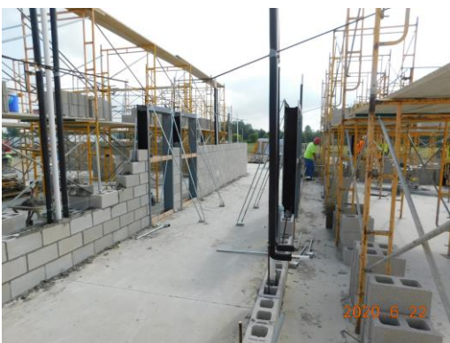
Unit D classroom wing CMU wall installation
