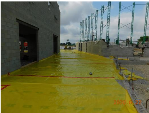
Concrete pour prep taking place in the corridors of the B/C connector
