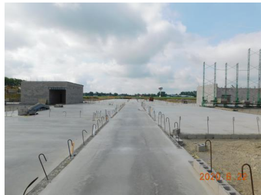
Concrete pour completed from last week in Unit C area
