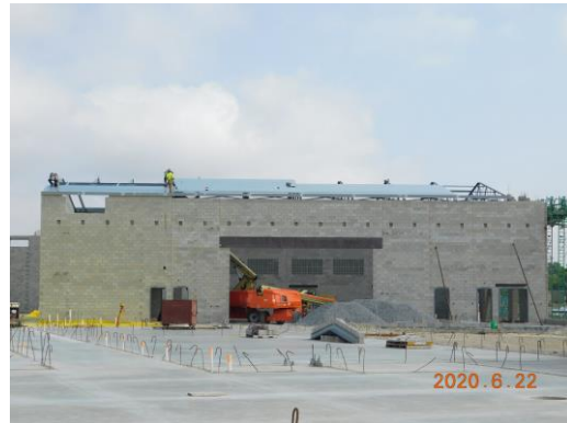
Decking installation taking place over the student dining area
