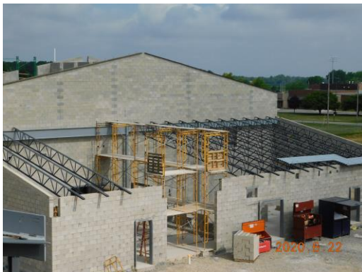
Bar Joists installed over the mechanical area of Unit A, East side of gym
