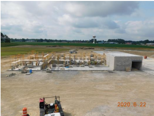
Unit D classroom wing CMU walls started
