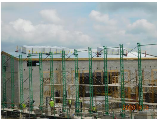
Roofing materials stored on student dining in preparation for dry in
