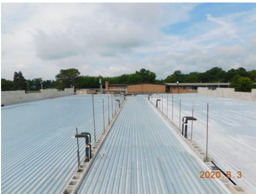
Unit C 2 nd floor classroom floor decking installed
