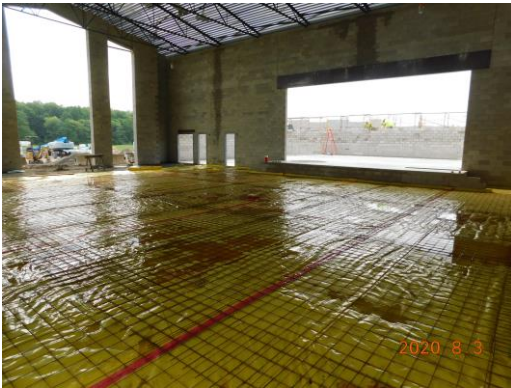
Floor prep taking place for student dining concrete pour
