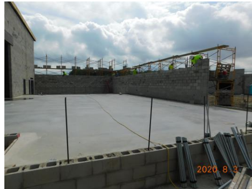
Stage walls being installed
