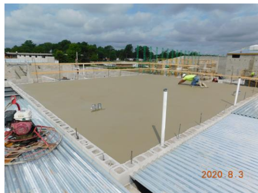
Unit D precast topping installed for mezzanine
