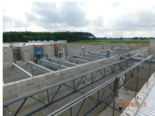
Steel installation on Unit C for 2 nd floor
