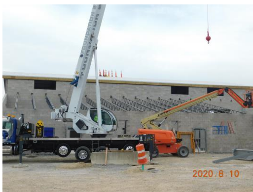
Bar joist installation on the kitchen area
