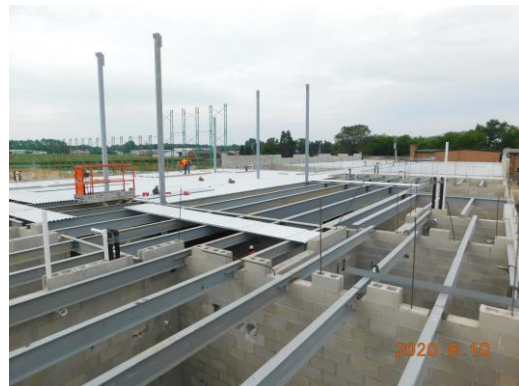
Steel for classroom hub viewing from the top
