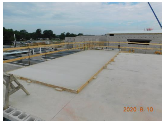
Unit D housekeeping pad for mezzanine equipment complete
