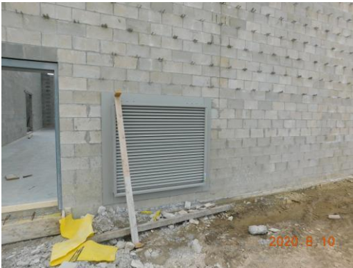
Louvers installed on the North wall of the gym in preparation for veneer
