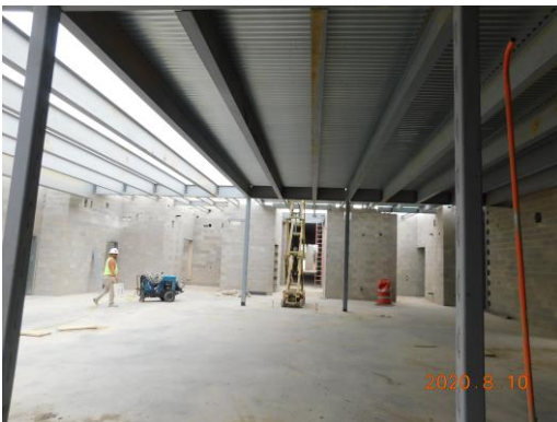
Steel and decking set in the classroom central hub area
