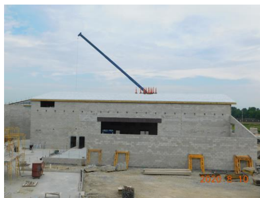
Roof dry in at the student dining is complete
