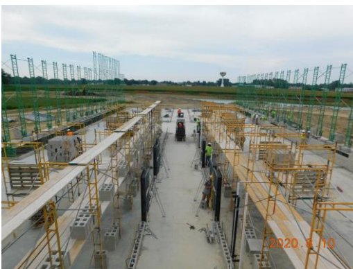
Unit E masonry bearing walls have started
