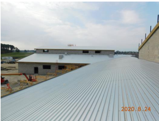
Decking installed at the Unit A to Unit B connector
