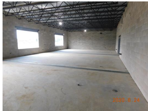
Unit C classroom wing with metal stud track in place in preparation of metal studs
