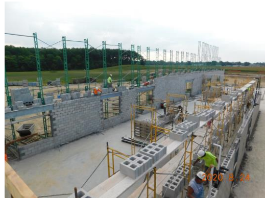
Unit E classroom wing wall installation continues, East side
