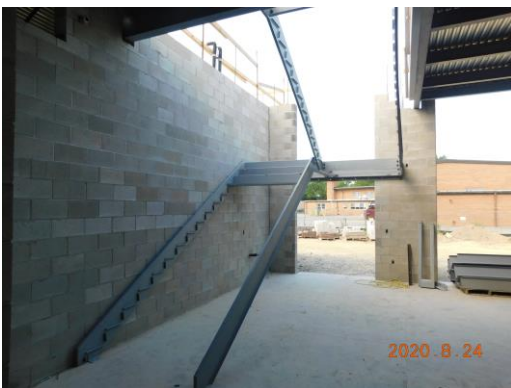
Unit C metal stairs have started to be installed West end of Unit C
