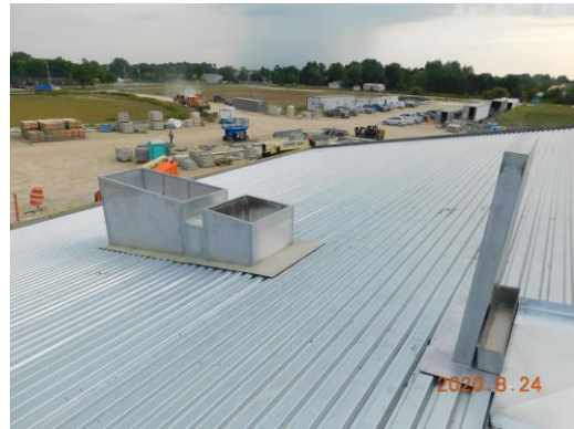
Unit B roof curbs above the kitchen area
