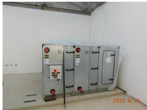
AHU piece set in the Unit A mezzanine
