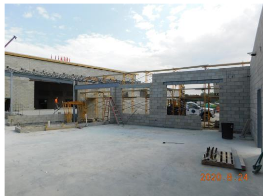
Masonry bearing wall installed south of the stage area
