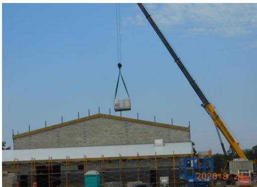
AHU pieces being swung into place in the Unit A mezzanine
