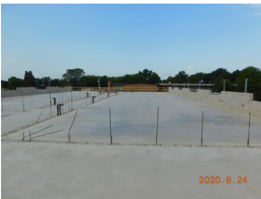
2 nd floor classroom wing concrete pour Unit C complete
