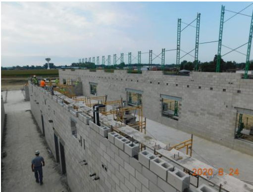
Unit E classroom wing wall installation continues, West side
