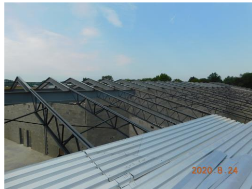
Steel and decking over Unit B corridor and media center
