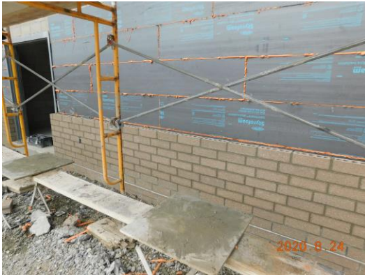
Veneer and cavity insulation installed on Unit A
