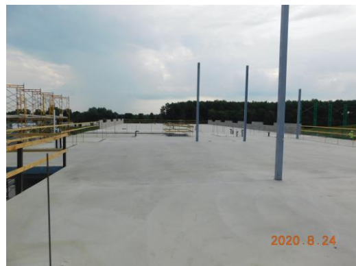
2 nd floor classroom wing concrete pour Unit D complete
