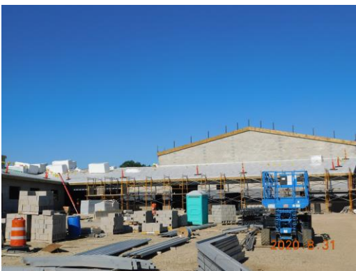
View of the low roof of A and part of B dried in
