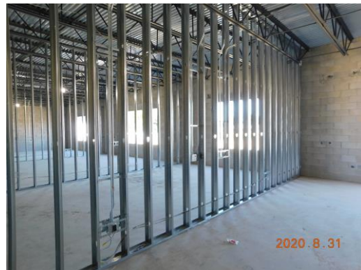
Unit C classroom wing metal studs showing some electrical rough in has started
