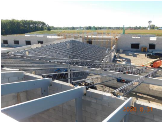
Steel work taking place in Unit B to the Unit C connector
