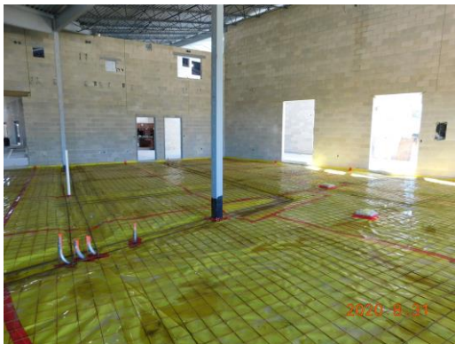
Media Center floor prep for concrete pour is taking place
