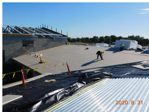
Unit B roof dry in taking place
