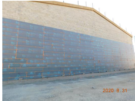
Cavity insulation installed on the west side of the gym
