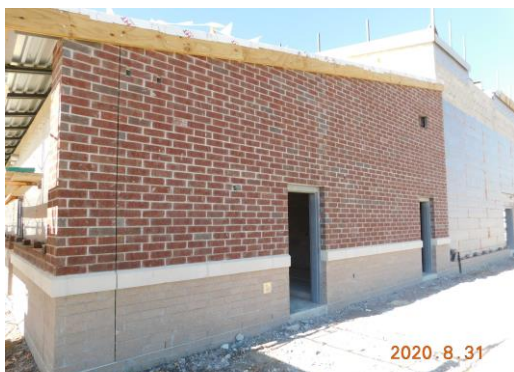
Veneer work taking place on Unit A
