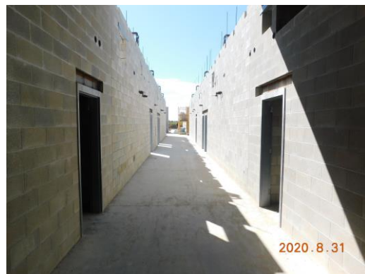
Unit E corridor walls completed to bearing height for 1 st floor
