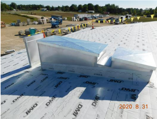
Roof and curb dry in above the kitchen area
