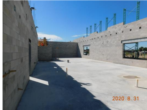
Unit E classroom bearing walls for 1 st floor almost complete
