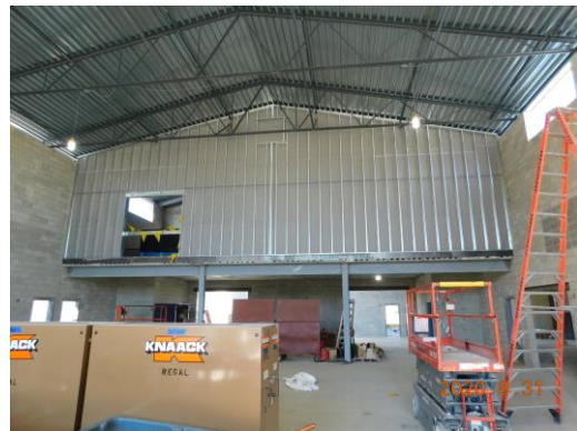
Metal stud and drywall installation taking place in the Unit B mezz. At student dining
