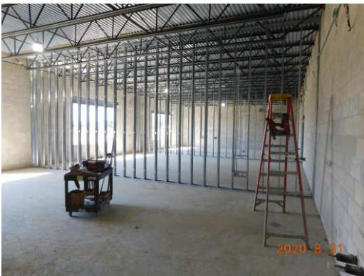
Metal stud installation has begun in the Unit C classroom wing (1 st floor)
