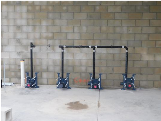
Restroom fixture carriers installation has started
