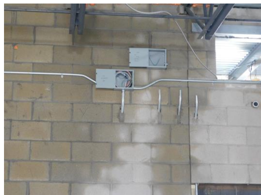
Electrical above ceiling rough in taking place in Unit C
