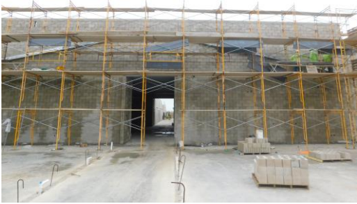
Scaffold set for veneer installation above roof at C hub area
