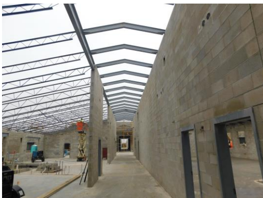
B to C corridor steel installation
