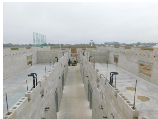
Unit E corridor walls completed to bearing on 1 st floor
