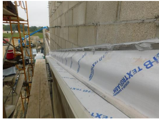
Flashing and term bar installation at the above roof area of Unit C hub
