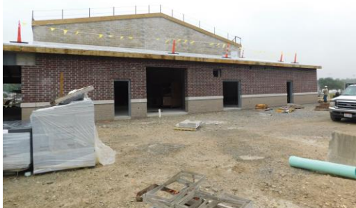
Veneer work on Unit A
