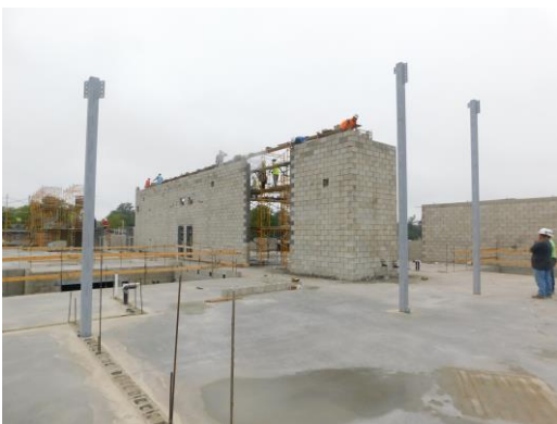
Unit C 2 nd floor masonry bearing walls being installed
