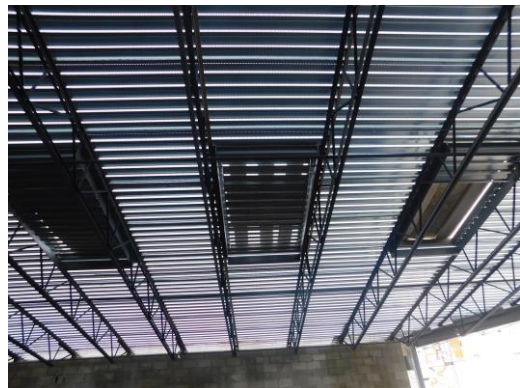
Smoke hatch layout and cut ins have started above the stage
