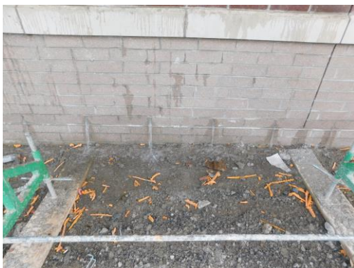
View of weep tests taking place and performing properly
