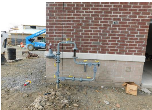
Gas line installation to the North side of Unit A
