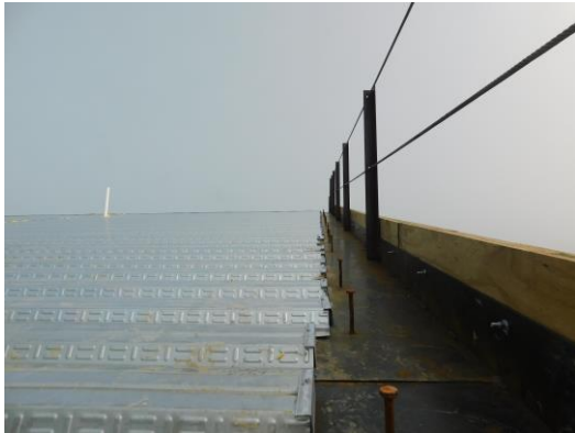
Studs installed up the East side rake wall of the gym roof for the concrete pour
