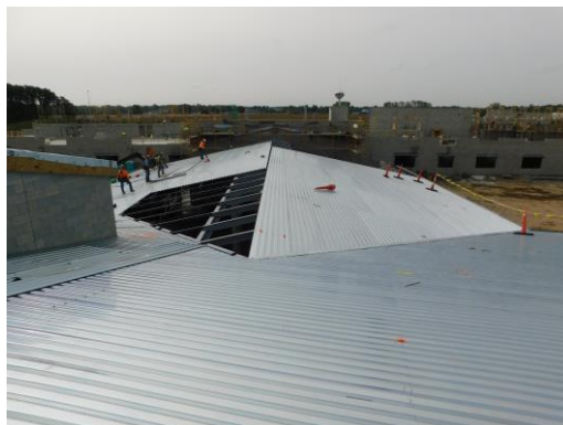
Roof decking being installed over the B/C connector
