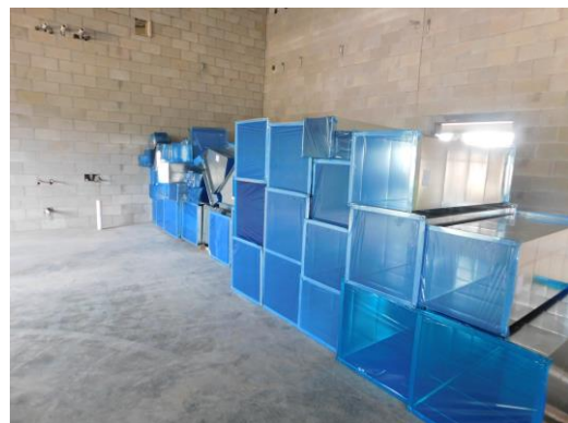
Duct work being brought to site and stored properly
