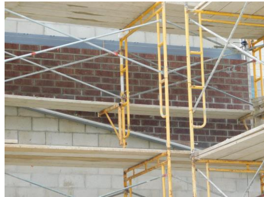
Veneer work is taking place on the B/C connector above the 1 st floor
