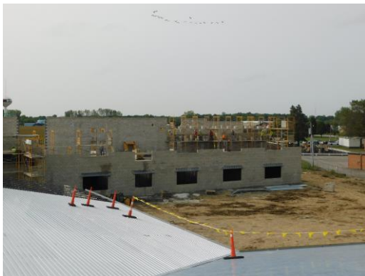
View of the classroom 2 nd floor area of Unit C masonry being installed
