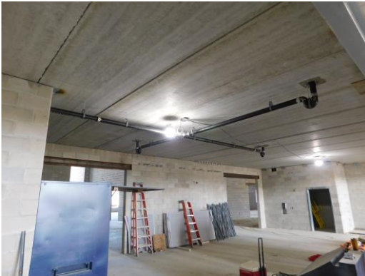
Drains are being installed below the mechanical mezzanine at the student dining
