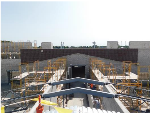
Veneer installed above the roof line at the B to C connector
