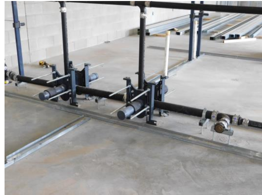
Restroom fixture carriers continue to be installed with wall clean out as well
