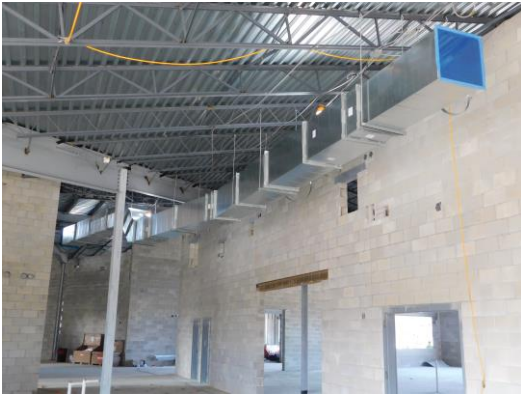
Ductwork installation started in the Unit B corridor
