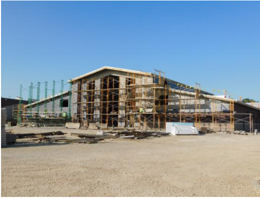
Veneer work taking place on the east side of the student dining
