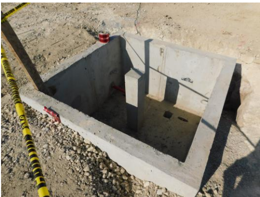
Vault for the transformer is installed
