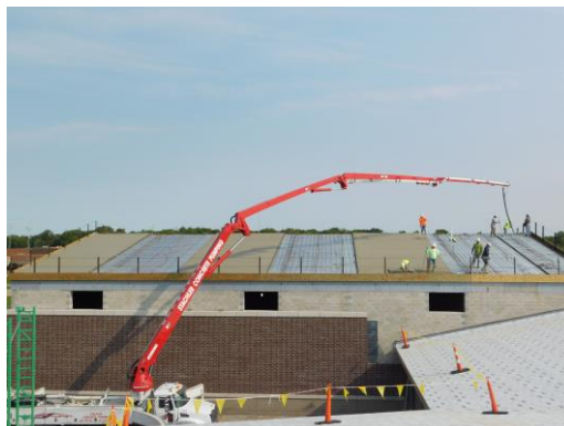
Day 1 of the gym concrete pour taking place
