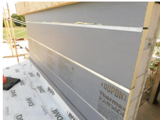
Insulation and Z furring for metal panels has started to be installed at the student dining
