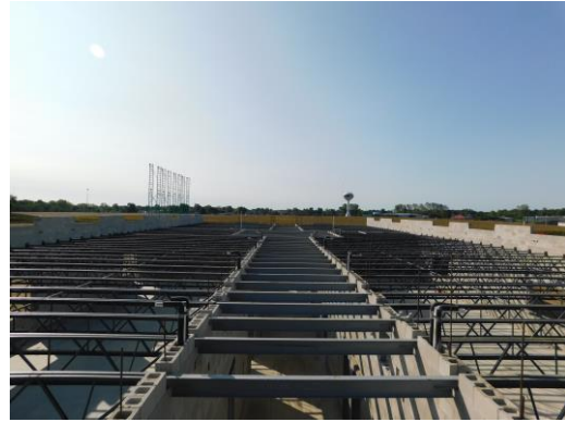
Unit E bar joists are installed ready for decking
