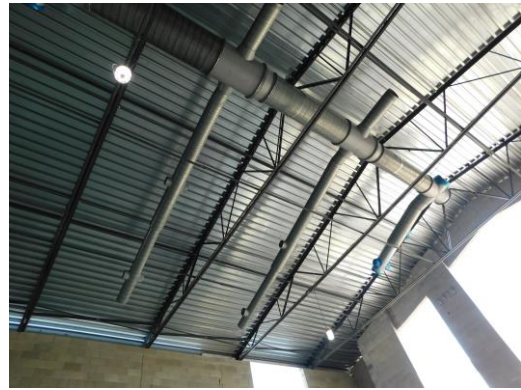
Round duct installation in the student dining has started
