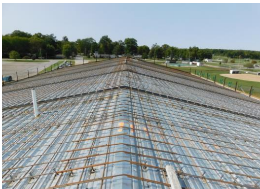
Rebar and Nelson studs installed on gym roof in preparation for concrete
