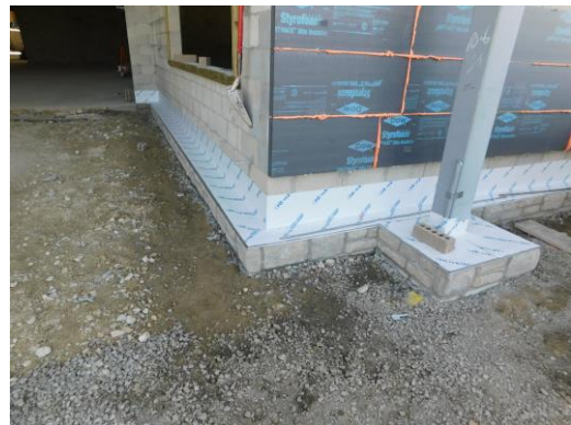
Cast stone installation has started at the main entrance
