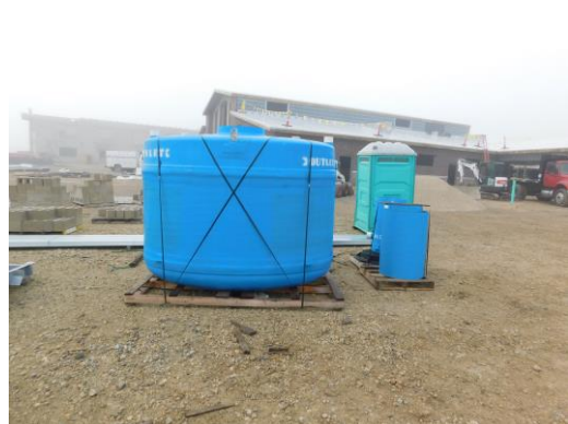
Grease interceptor is on site and ready for installation outside the kitchen this week
