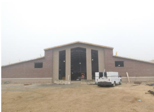
Veneer complete on the East side of the student dining
