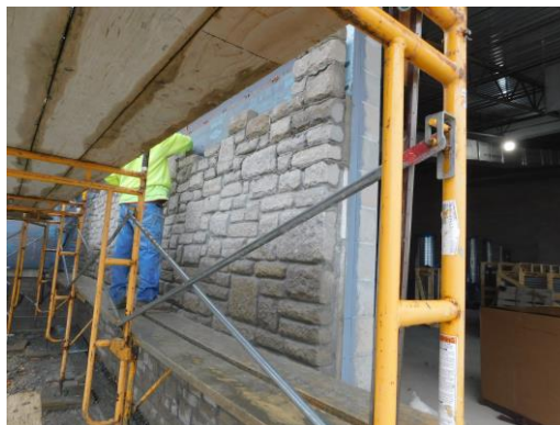
Stone veneer installation continues on the West side by the main entrance
