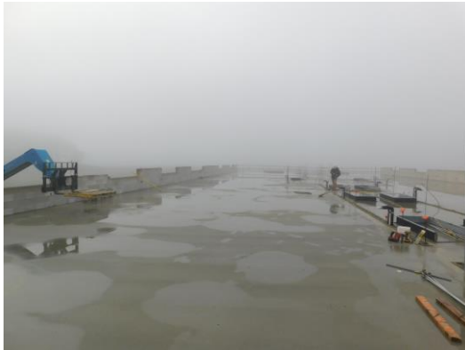
Concrete pour for the 2 nd floor units E and F is complete
