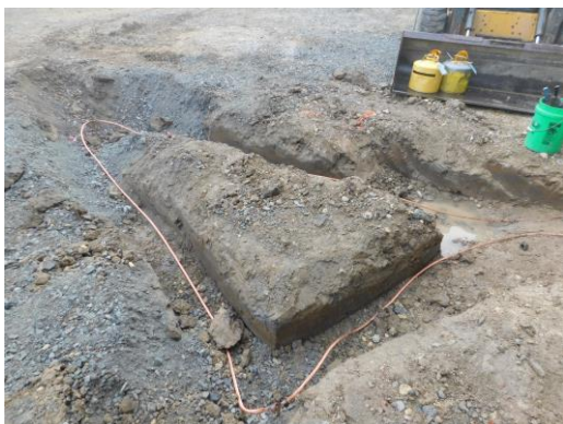
Electrical grounding grid installation has started
