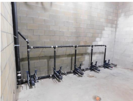
Restroom carriers and vent piping installed for one of the group restrooms
