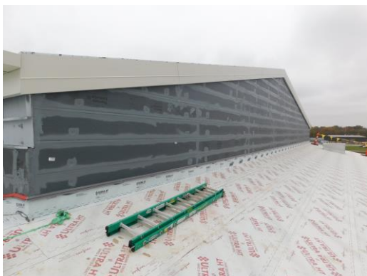
Metal panel insulation joints sealed prior to metal panel install
