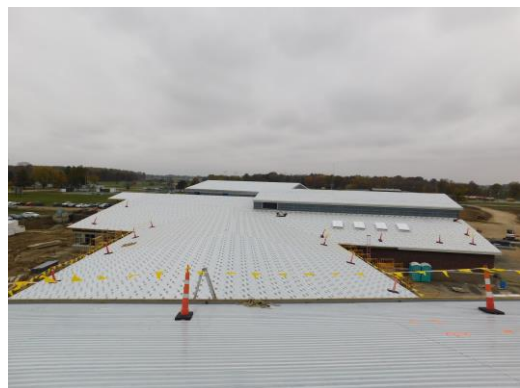
View of Units A and B from Unit C rooftop
