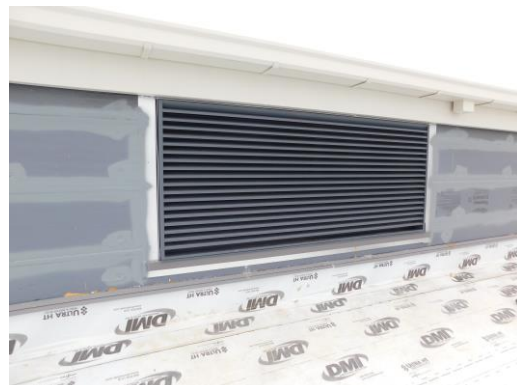
Louvers installed over student dining area
