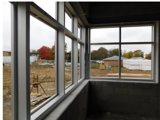
Window installation in Unit B admin area
