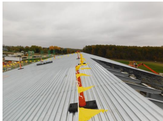
Unit D decking from the top
