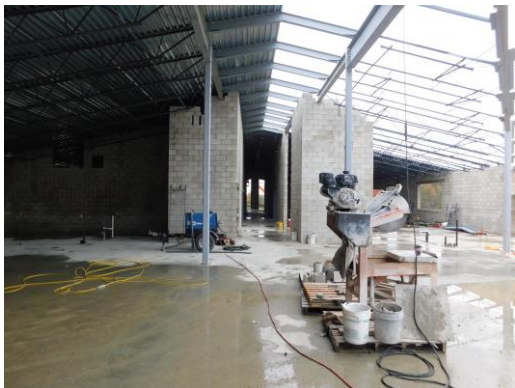
Steel and decking being installed on Unit D
