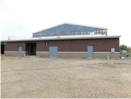
Unit A doors installed and brick washed
