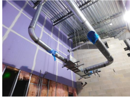
Mechanical equipment being installed in the Admin area of Unit B
