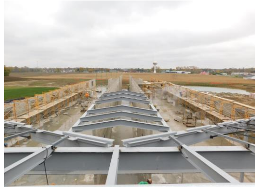
View of Units E and F from the rooftop of Unit C
