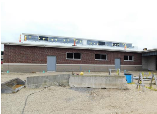
Brick cleaning and window installation has started on Unit B
