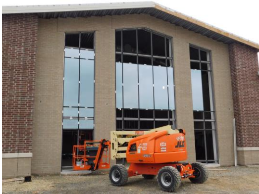
Curtain wall glazing has started at the student dining
