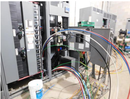
Electrical wiring being pulled as part of the switchgear wiring
