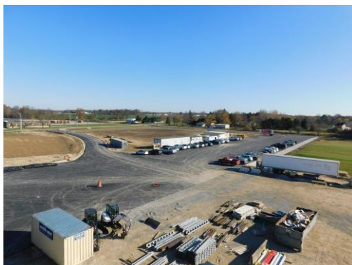
Base course of asphalt is installed on the east side of the site
