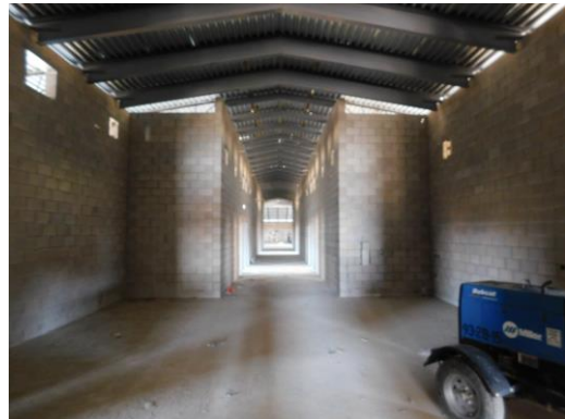
View down the 2 nd floor Unit E corridor looking North
