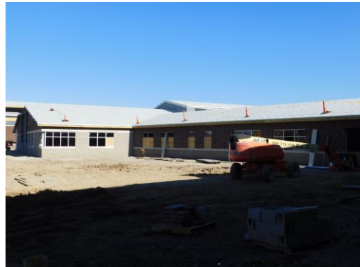
Veneer and window installation on the West side of Unit B
