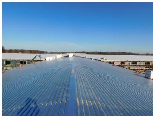
Decking is installed over Units E and F
