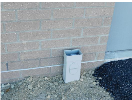
Downspout boots installed around areas that received asphalt
