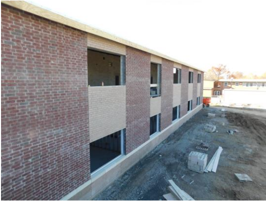
Veneer installed on the North side of Unit C
