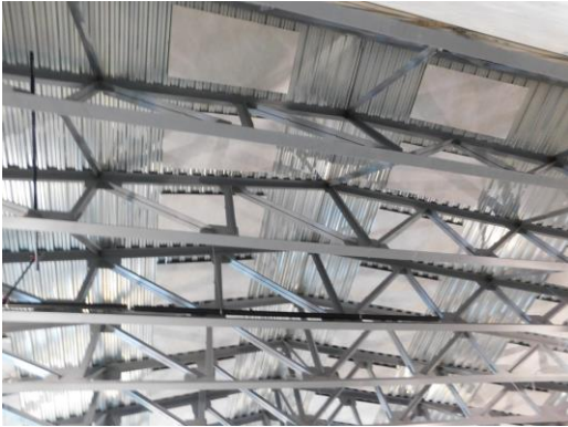
Tectum panels installed on the gym roof as part of the acoustical dampening
