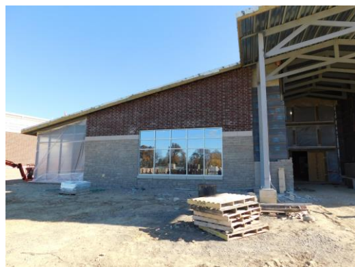
Window installation at the media center on the west side of the building
