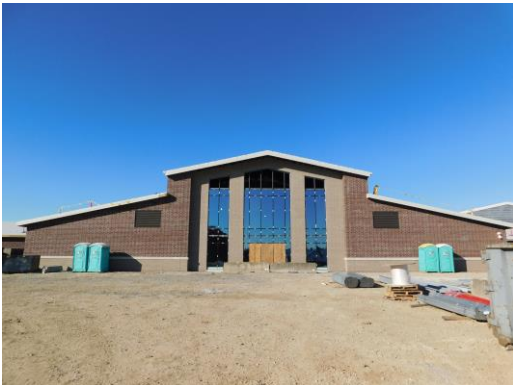
Window installation on the East side of the student dining
