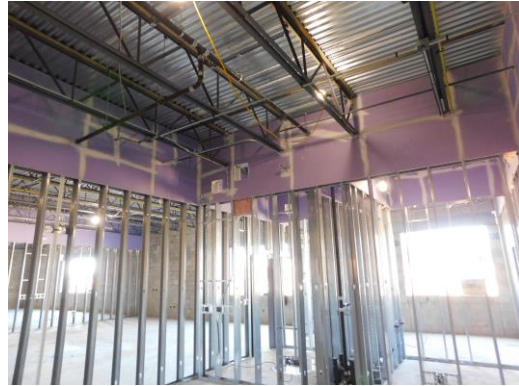
Drywall top installation in Unit E
