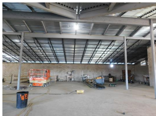
View of the 2 nd floor central hub area
