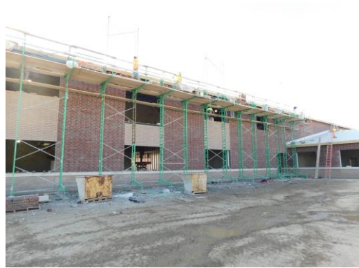
Veneer installation taking place on the North side of Unit D
