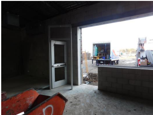
Exterior door installation being started from the art room
