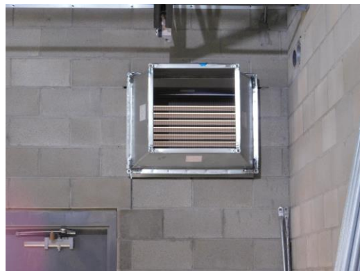
Louver installation in Unit A
