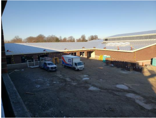
Veneer installed on the East side of Unit B and window install taking place
