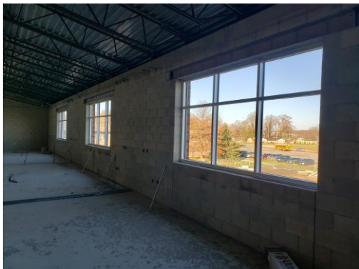
Window installation taking place on Unit C 2 nd floor taking place
