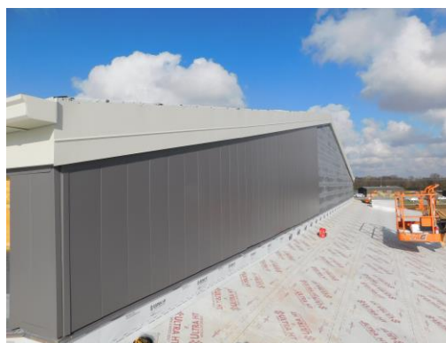
Metal wall panel installation is taking place on the gym
