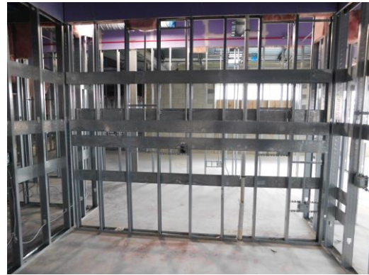
In-wall blocking taking place in the admin area
