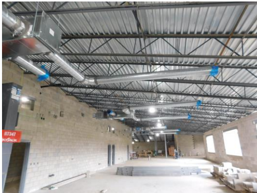
HVAC above ceiling rough in taking place in the 2 nd floor classroom wings
