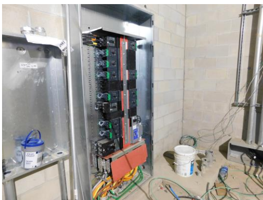
Wire being pulled to panels throughout the building
