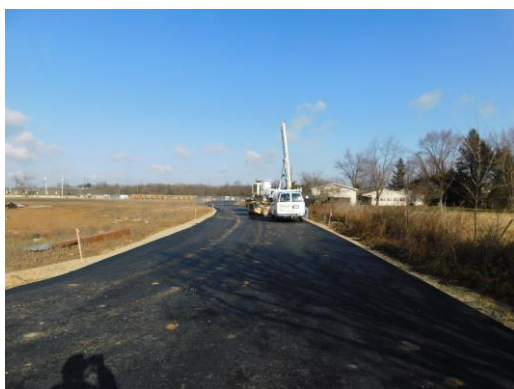
Light pole bases are being drilled for placement
