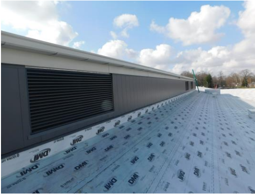
Metal wall panel installation over the student dining area
