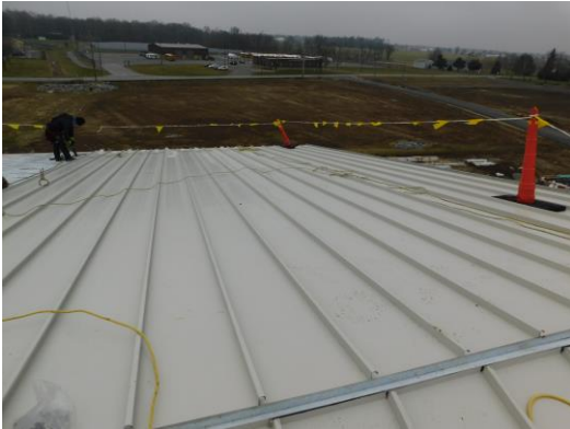
North side gym panel installation has started
