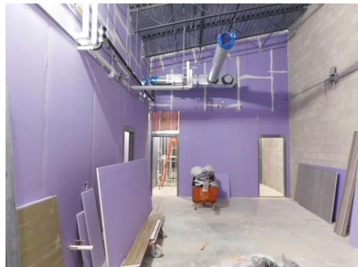
Drywall continues in the Admin area
