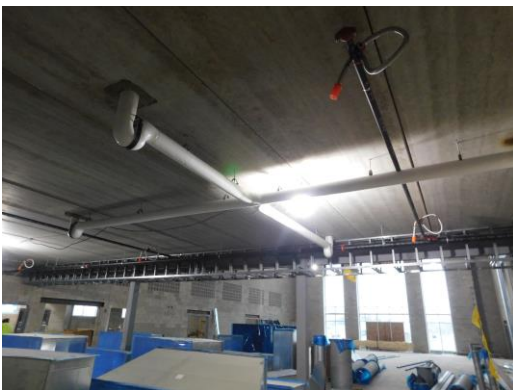
Drain pipe insulation continues in Unit B
