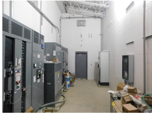
Block Fill and paint in the main electrical room
