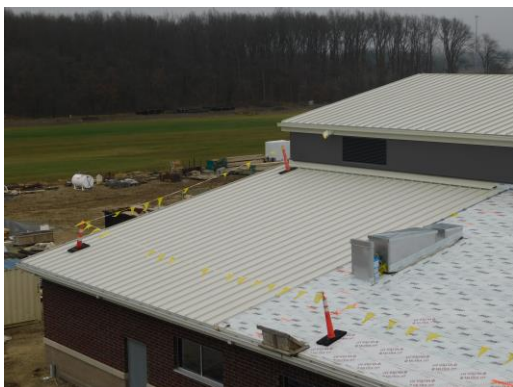
Metal roof panels installation over the kitchen area
