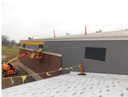
Metal wall panels continue to be installed
