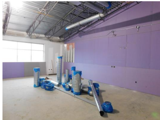
Drywall installation is taking place in the 2 nd floor Unit D classrooms
