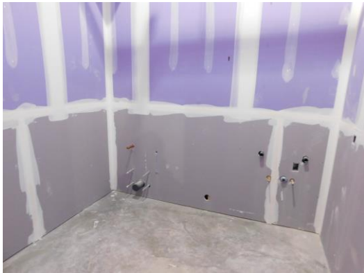
Drywall mud in restroom of admin area is taking place as well
