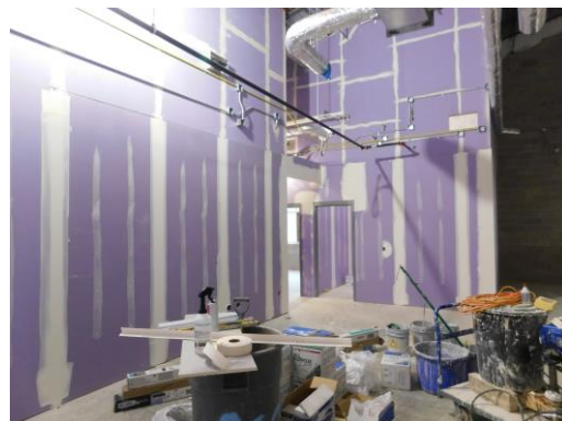
Drywall mud has started in the admin area
