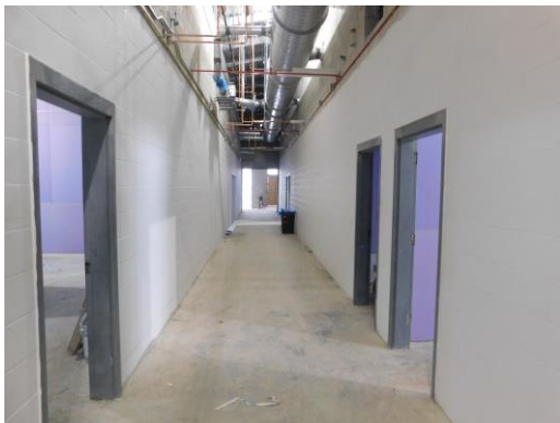
Block fill has started in the 2 nd floor Unit C and D classroom wings
