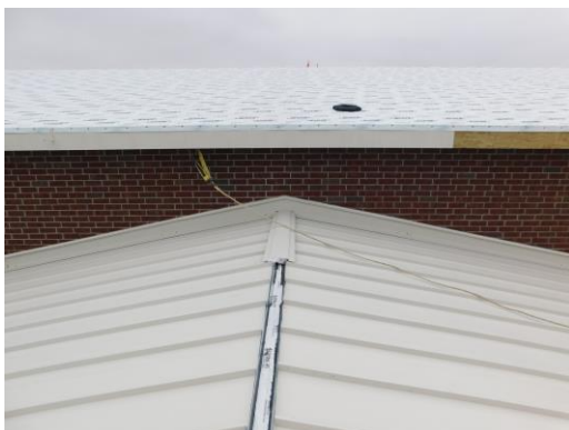
Metal roof panels installation over the Unit B/C connector
