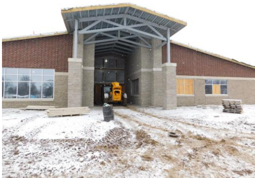
Main entry stone veneer complete
