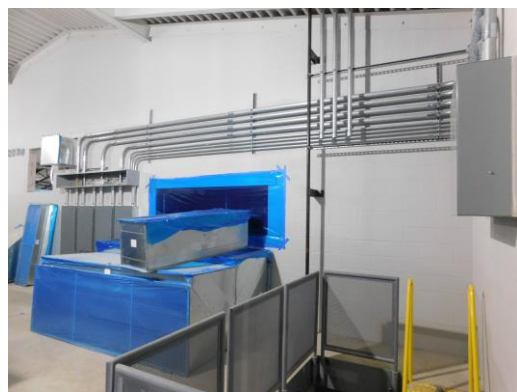
Electrical and Ductwork continues on the Unit B mechanical mezzanine
