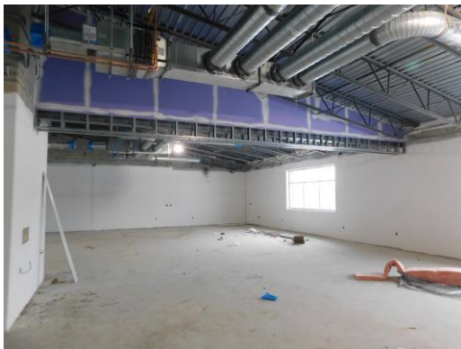
Drywall and block fill installed for 2 nd floor classroom with operable wall
