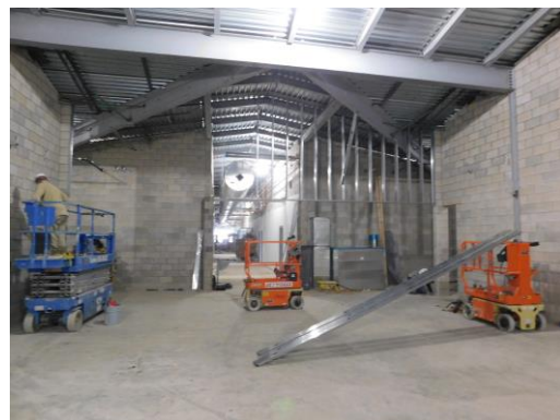
Unit C hub classroom started on 2 nd floor
