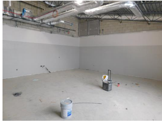
2 nd coat of paint being installed on 2 nd floor Unit C classrooms
