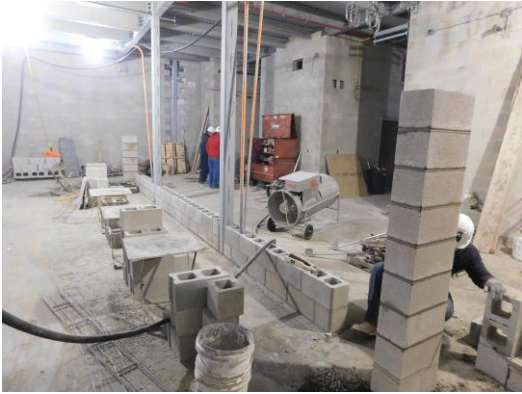
Unit C hub classroom walls being started on 1 st floor
