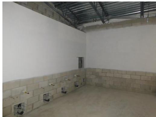
Block fill in one of the group restrooms
