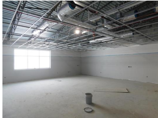
Grid installation continues on 2 nd floor
