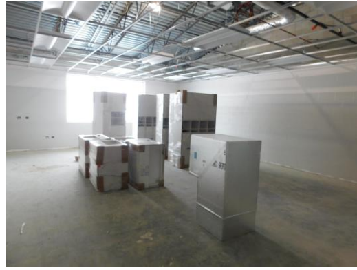
Casework is being delivered and placed in rooms for installation on 2 nd floor
