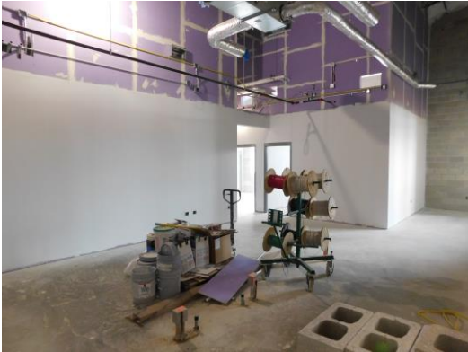
Paint has started at the main entry reception area of the admin. office
