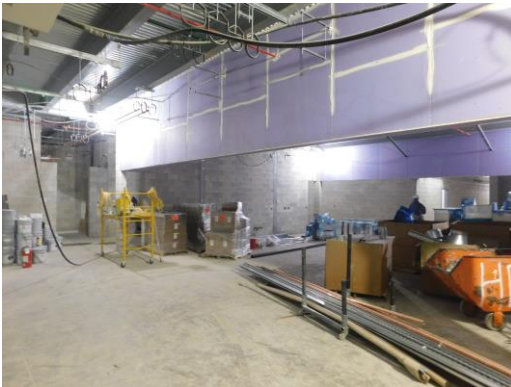
Work continues at the 1 st floor Unit C hub classroom area
