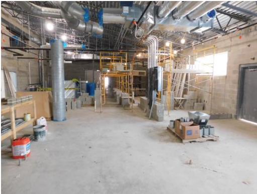
MEP work taking place in the kitchen
