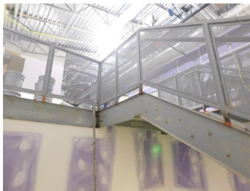
Stair railings are being installed
