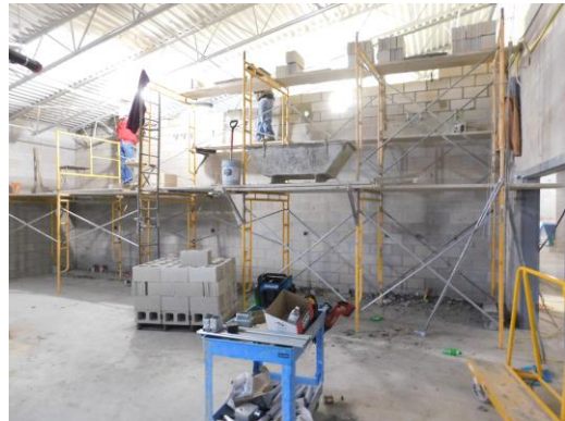
Interior CMU continues in Unit B
