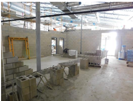
Interior walls being installed at the media center area continues
