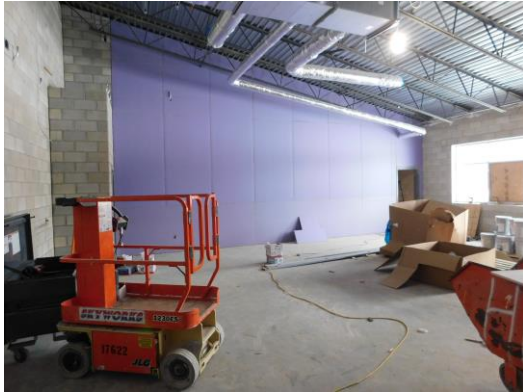
Drywall wall installed to separate the music rooms
