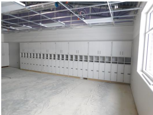
More casework installation in Unit C 2 nd floor
