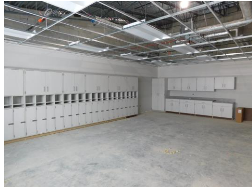
Casework installation has started on the 2 nd floor of unit C
