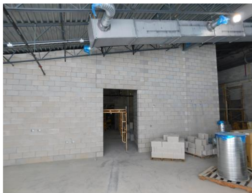
Masonry walls for the media center completed
