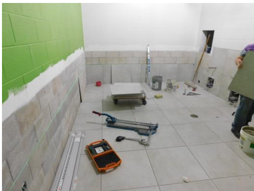
Ceramic tile being installed on the restroom wall on the 2 nd floor
