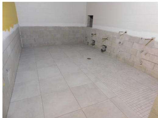
Ceramic tile installed on the restroom floor of a 2 nd floor boys restroom
