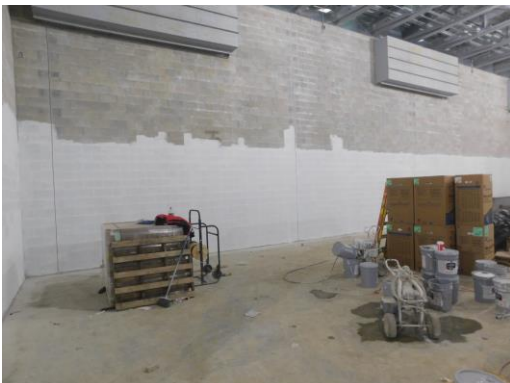
Block fill paint has started on the gym walls.
