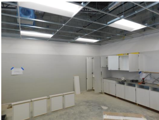
Casework installation has started in Unit D 2 nd floor
