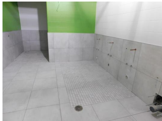
Restroom wall and floor tile ready for grout in group restroom on 2 nd floor
