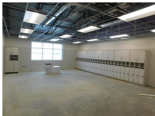
Room with casework and permanent lighting installed and operational
