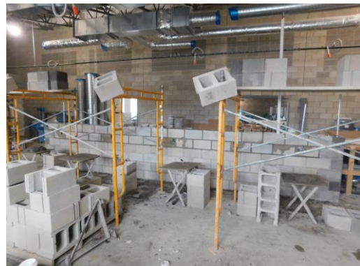
Masonry walls continue in the kitchen area
