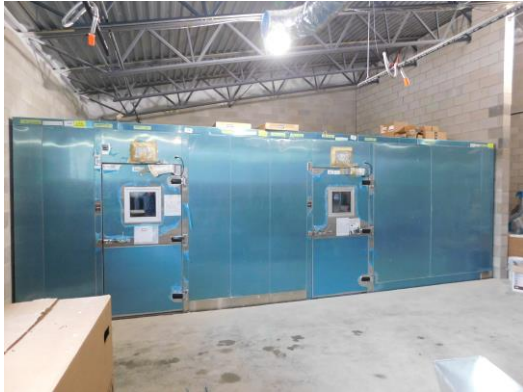
Cooler/Freezer installation in the kitchen area
