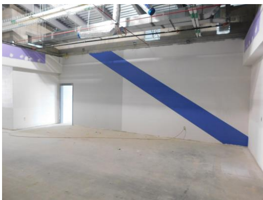
Accent paint striping has started in Unit E 2 nd floor ELA area
