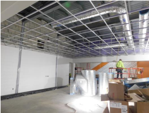
Grid installation has taken place in the 2 nd floor hub classroom
