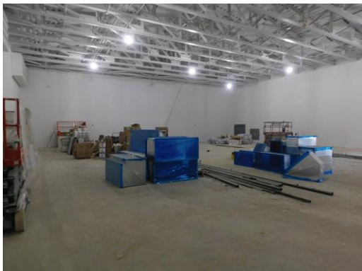
Paint continues in the gym
