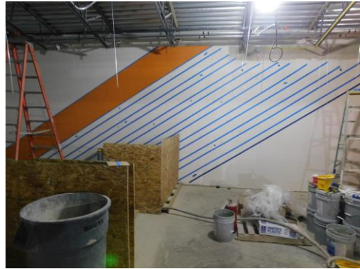
Accent striping and layout prep is taking place on the 2 nd floor
