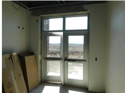
Exterior door installation has taken place at the south end of Unit E
