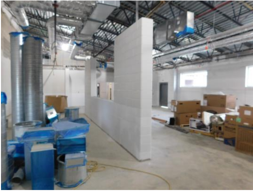
Painting in the kitchen has started
