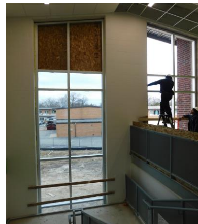
Clearstory windows being installed In Unit C
