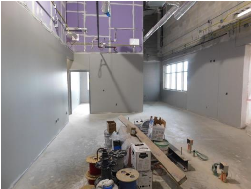
Final paint color being installed in the administration area
