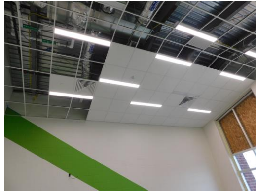
Ceiling grid and pads installed above the stairwell Unit C
