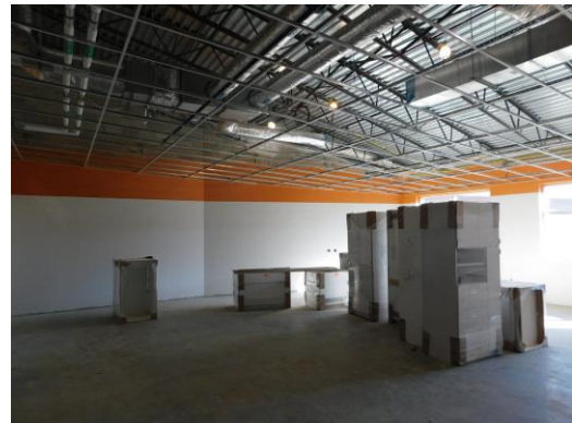
Ceiling grid installation has taken place in one of the art rooms
