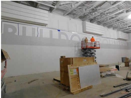
Stenciling is being put in place on the gym walls in preparation for painting
