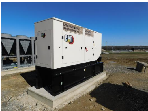
Generator has been set in place on the north side of the building
