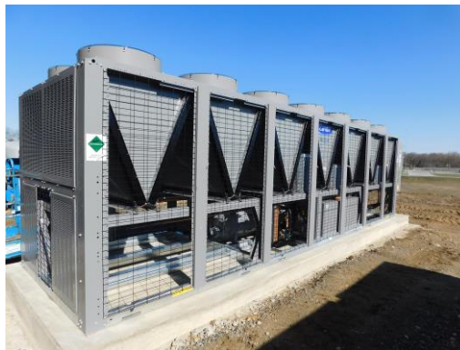
Chiller has been set on the north side of the building
