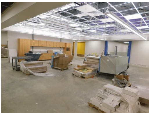
Lighting is complete on the 2 nd floor C "hub" classroom
