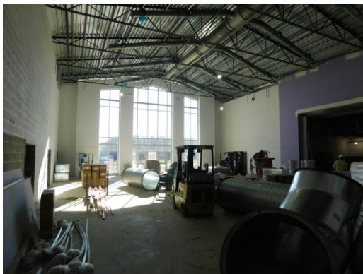
Paint work continues in the student dining
