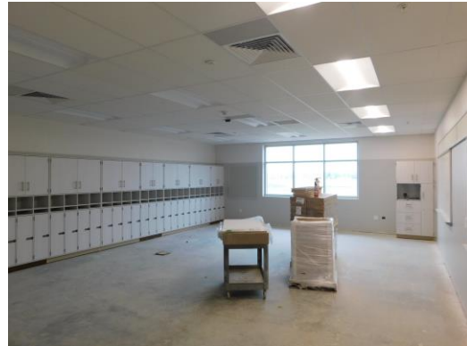
Ceiling pad installation in 2 nd floor classroom
