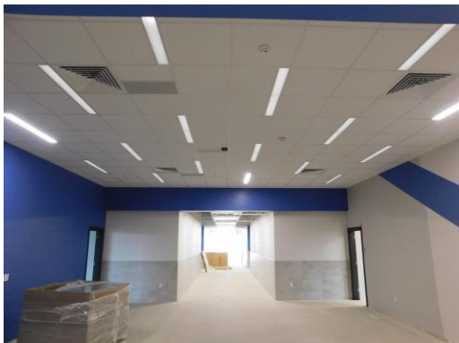
Ceiling tile installation in the Unit E ELA
