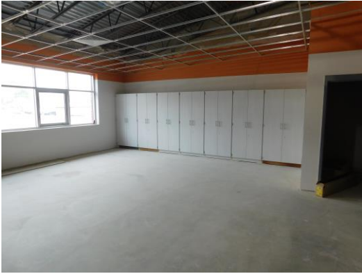
Casework installation in the art room has started to be installed
