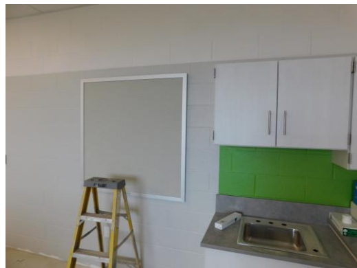
Tack board installation has started on the 2 nd floor
