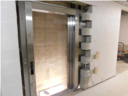
Elevator installation has started
