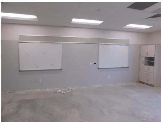
Marker board installation has started on the 2 nd floor
