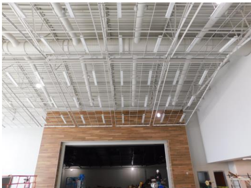
Ceiling grid installation taking place in the student dining
