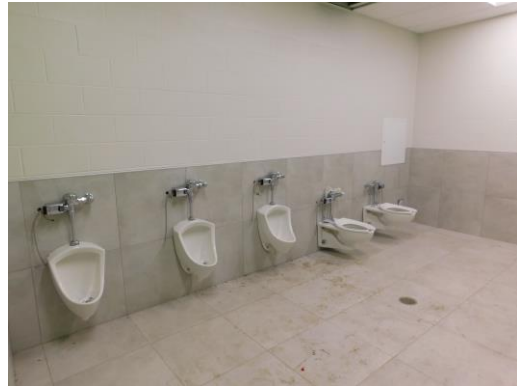
Restroom fixture installation has started in the group restrooms
