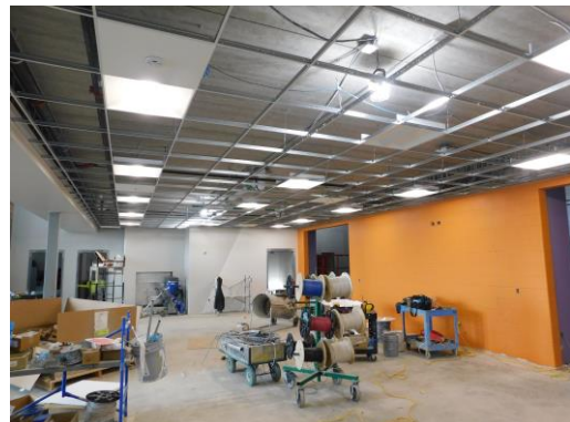
Ceiling grid installation in west end of student dining
