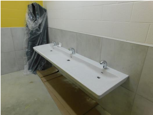
Restroom sink installation has started outside the group restroom areas
