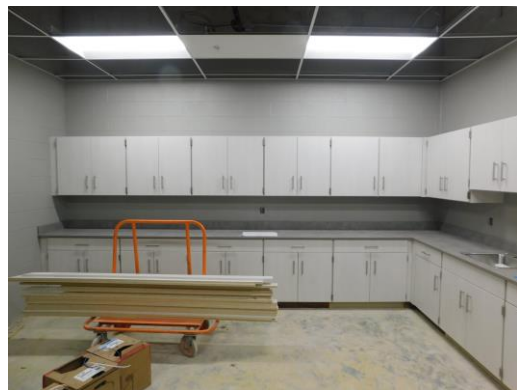
Casework installation in one of the teacher work rooms
