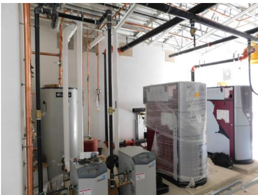
Main mechanical room equipment being set and piped in
