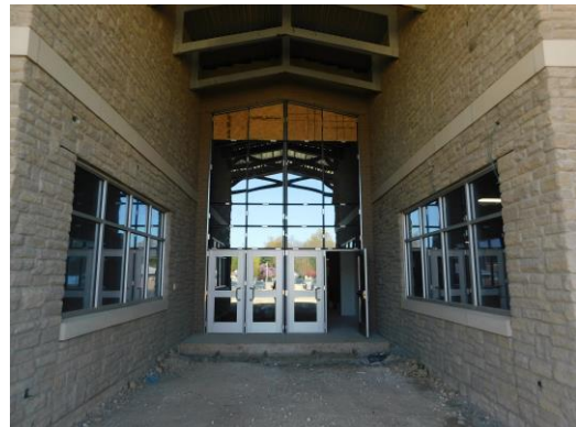
Main entry storefront installation continues
