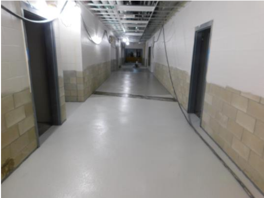
Terrazzo pours taking place in the connector corridor
