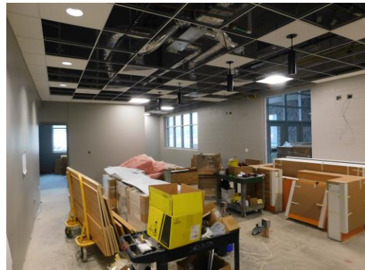
Ceiling pad installation has started in the admin area
