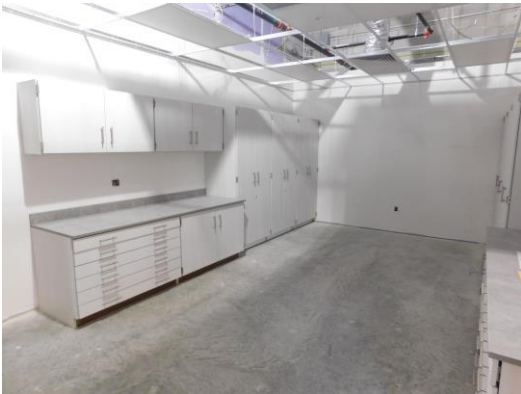
Casework installation in the art kiln room has taken place
