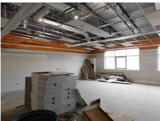
Lighting and ceiling pad installation started in the art room
