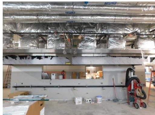
Kitchen hood duct insulation is completed
