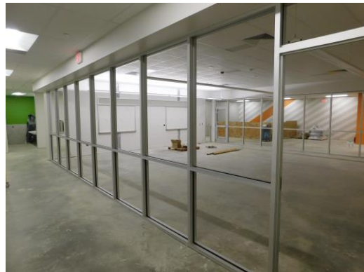
Framing for the science/tech sign out room is taking place
