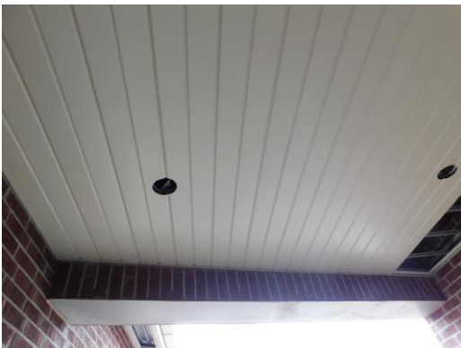
Soffit installation over one of the canopy entrances is taking place
