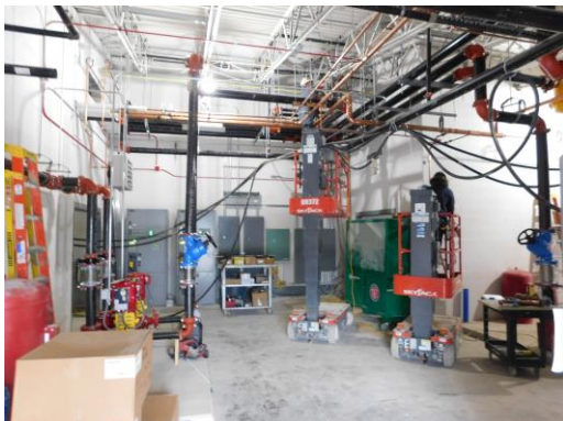
Work in the main mechanical room continues
