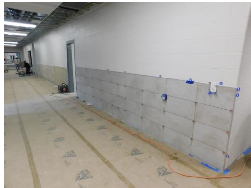
Wall tile installation continues on the main corridor
