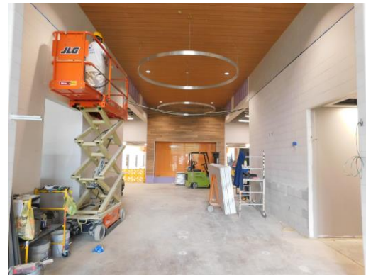
Paint and ceiling installation in the main entryway
