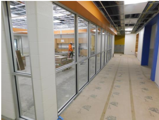
Window framing for the 1 st floor science lab sign out room is installed
