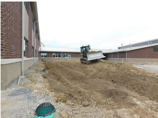
Playground prep work has started
