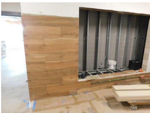
Wall tile installation outside of the art rooms for the display case
