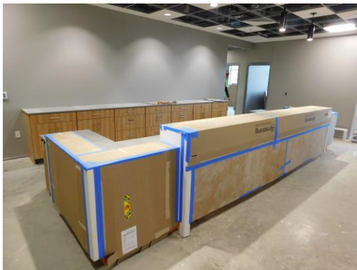
Casework installation in the main office reception area
