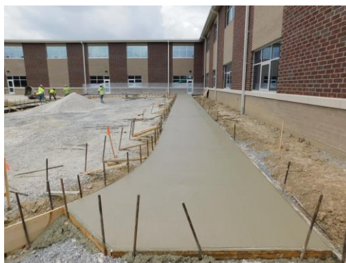
Site concrete pours taking place on the east side
