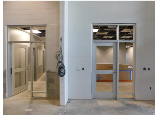
Entry door installation to the admin reception area
