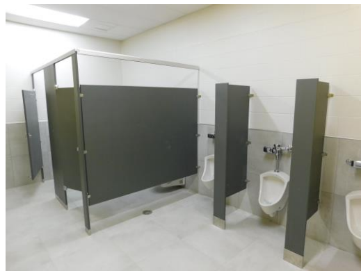
Toilet partition installation in one of the boys group restrooms
