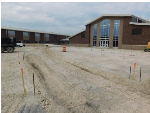
Playground prep work continues
