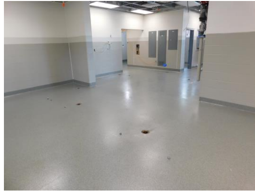
Epoxy flooring installed in the kitchen areas
