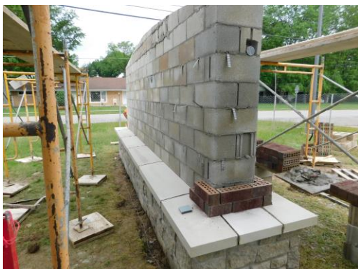
Masonry work taking place on the main entry sign
