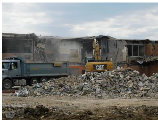
Demo of the existing building is taking place
