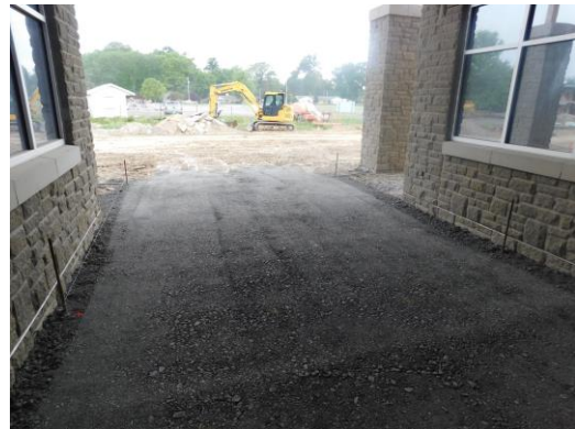
Stone prep for concrete pours at main entry
