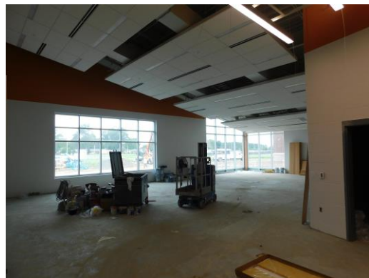
Ceiling installed in the media center
