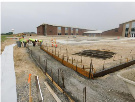
More concrete pours taking place today for the playground area
