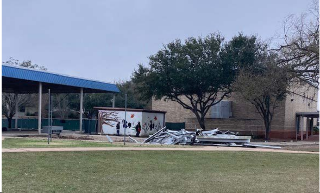
Courtyard canopy demolition
