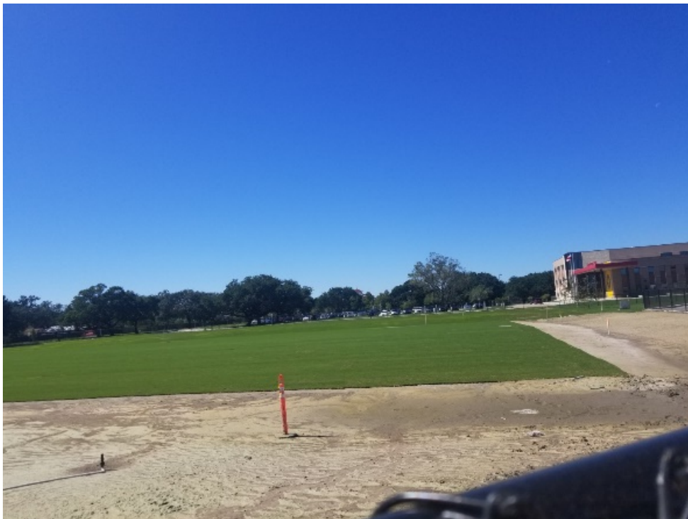
Sod at front Practice Field
