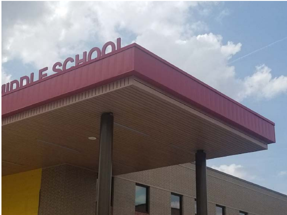
Entry Canopy Complete
