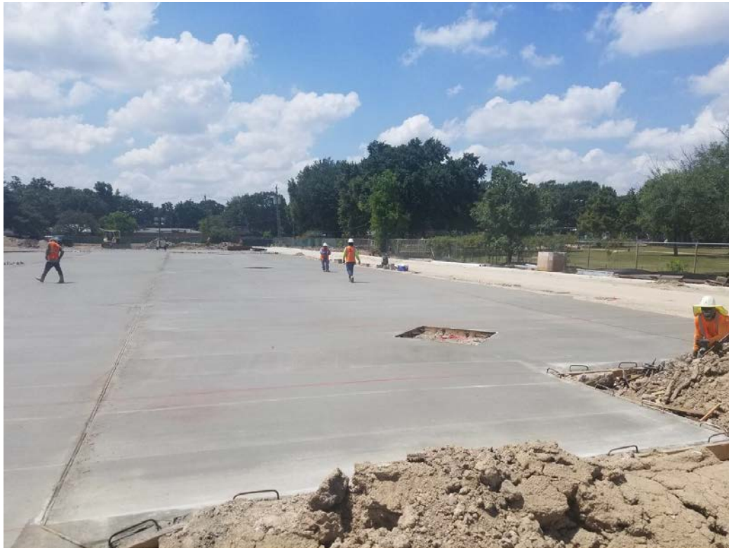
Front parking concrete poured
