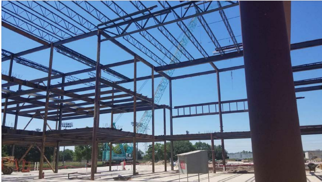
Steel Erection Area A – June 12th
