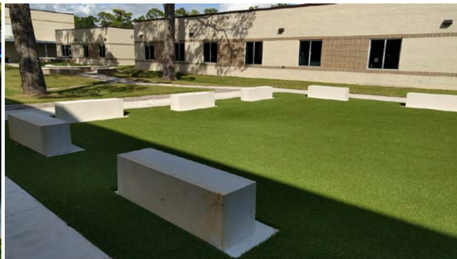
Limestone Benches Installed
