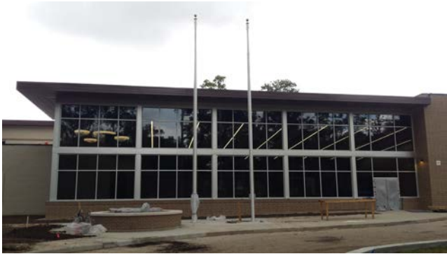
Library- Exterior Progress
