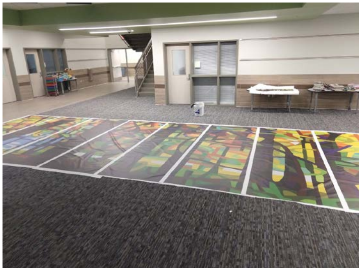
Wall Graphics Installation In Progress
