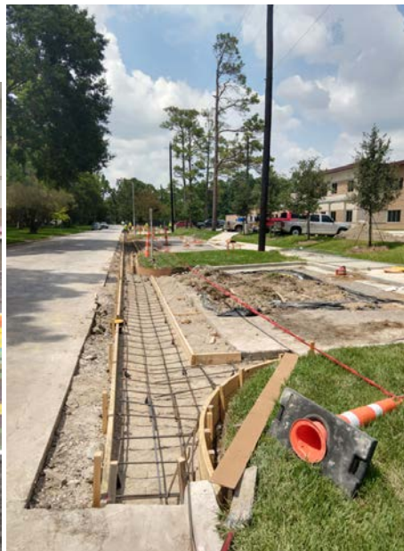
Wade Hampton Repairs in Progress
