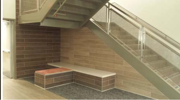
Solid Surface installation at T-Bench Pending
