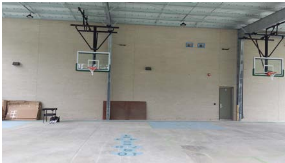
Basketball Goals Installed
