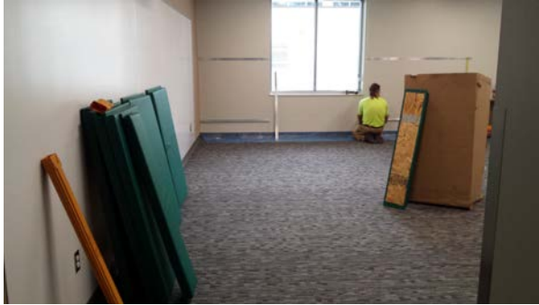
Wall Pads at Motor Skills- Progress
