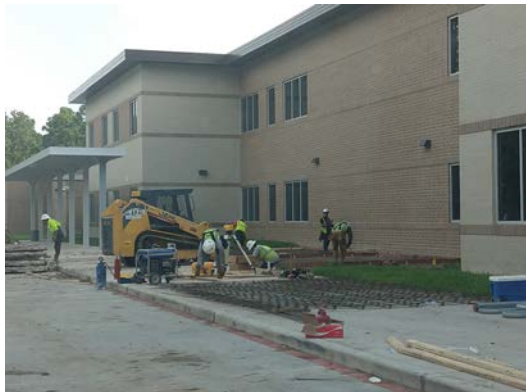
Bike Racks- Installation in Progress
