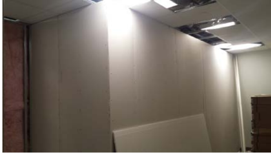
Added Speech Rooms In Progress
