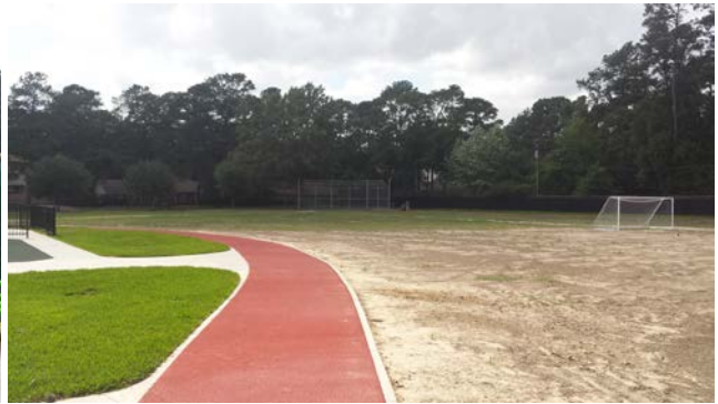
Track Surface Installed
