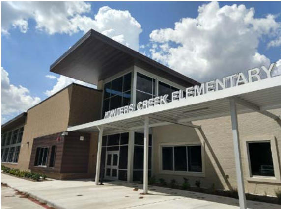
Canopy Letters Installed
