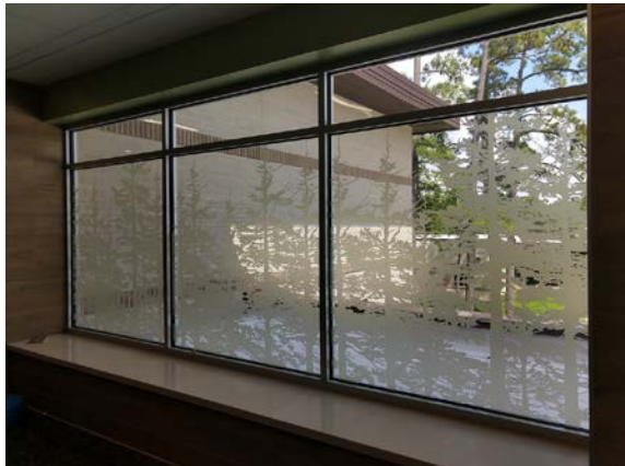
Window Film Installed (At Area D2)
