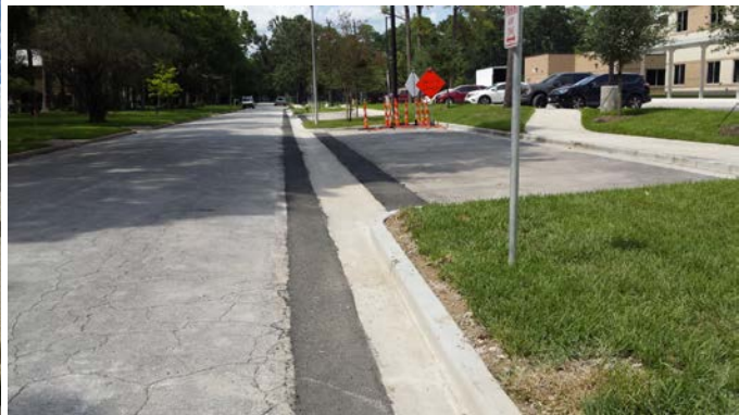
Wade Hampton Repairs Completed
