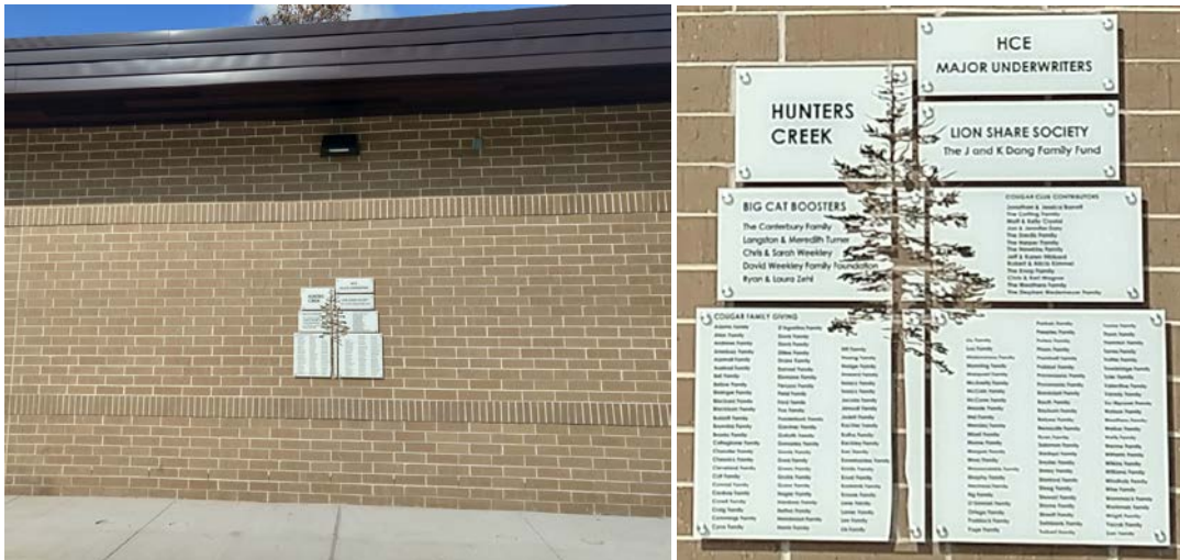
Donor Plaque Installation, Wall Pack light centered Above
