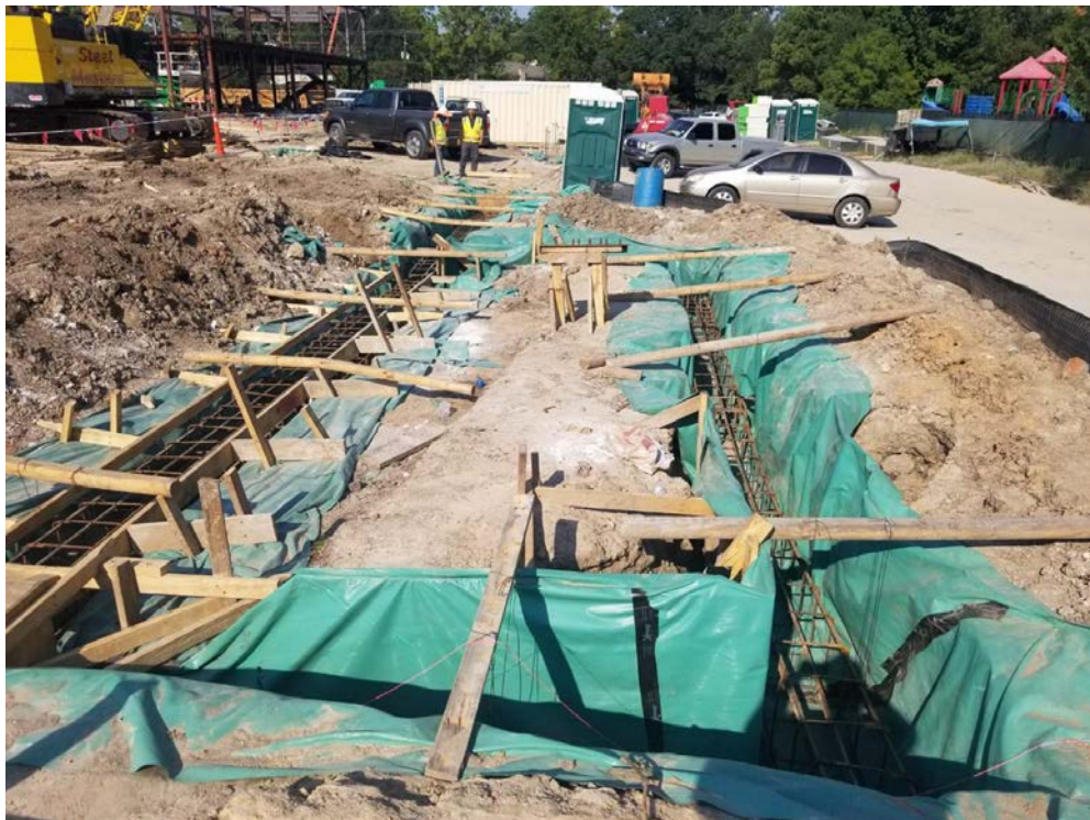
Forming Foundation for Outdoor Storage Building
