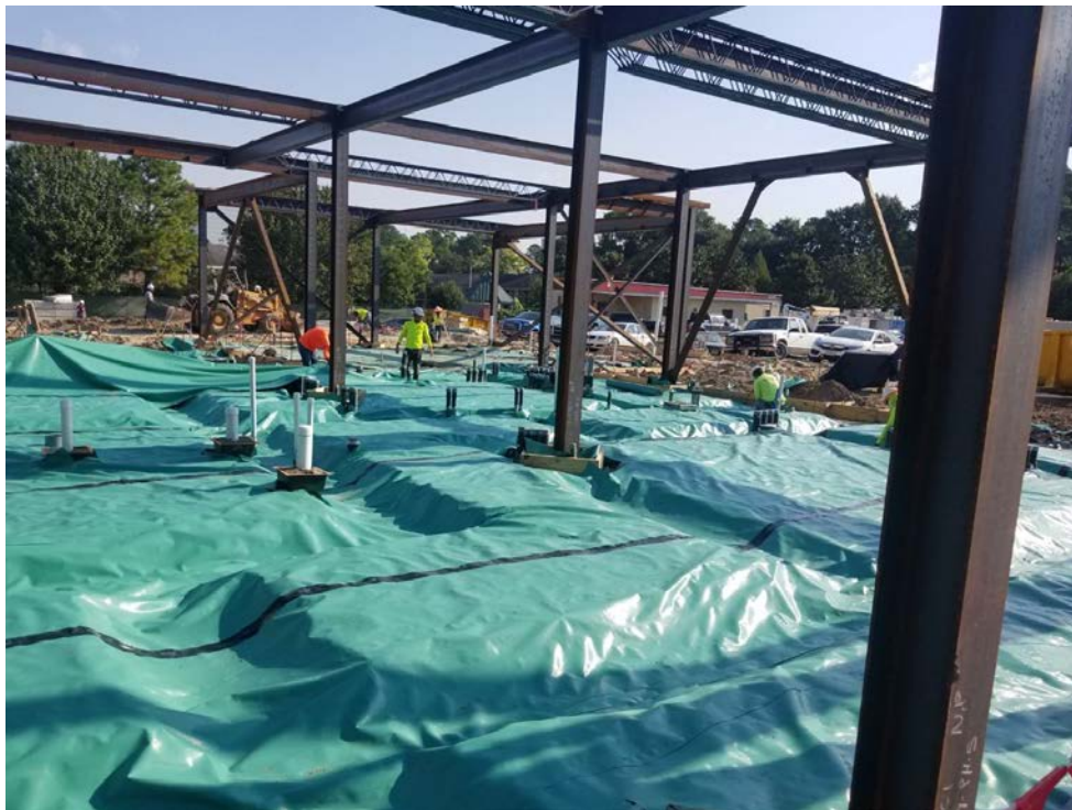
Slab Prep at Kitchen
