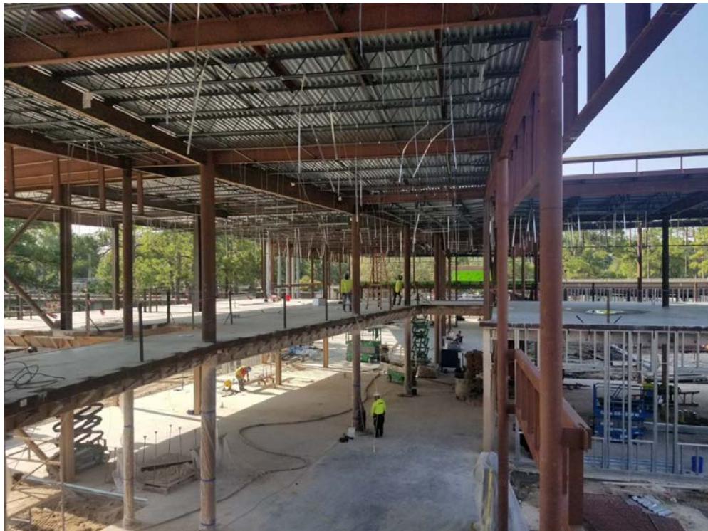
2 nd Floor Interior View
