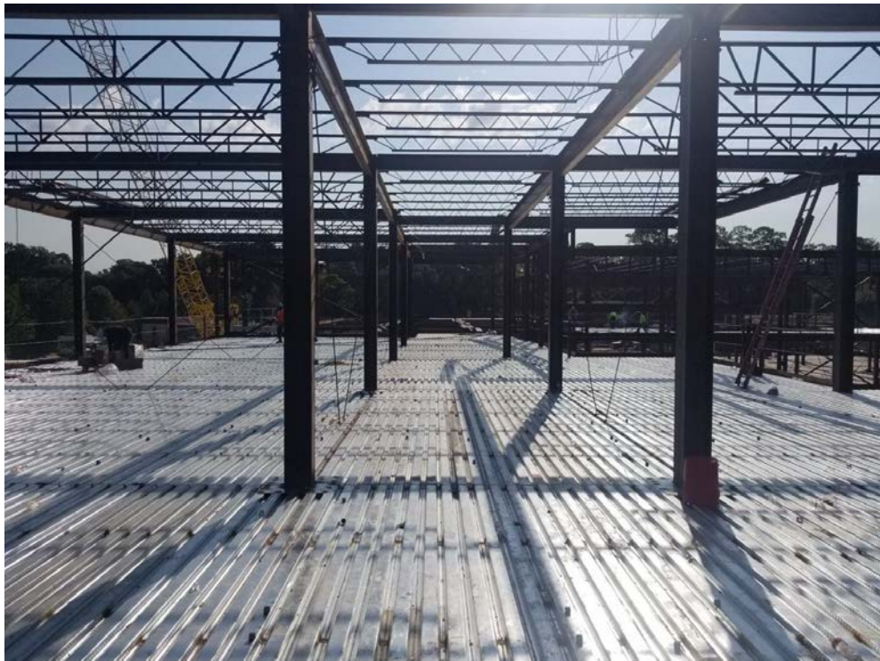
Area D 2 nd Floor Decking
