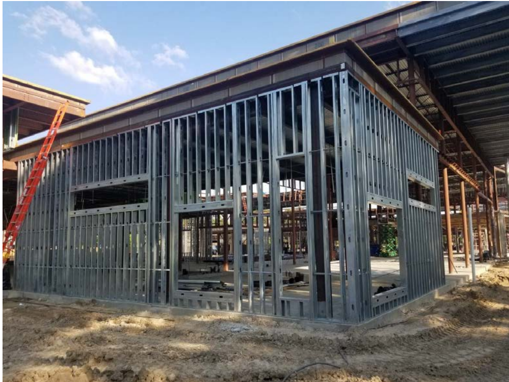
Exterior Framing at Multi Purpose Room
