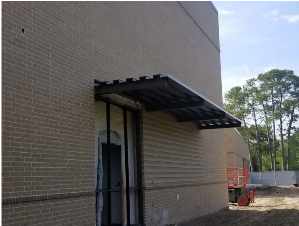
Avadek Canopies at West Elevation
