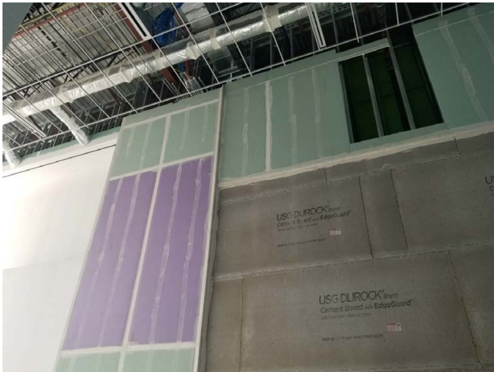
Framing at Dining Graphics Wall
