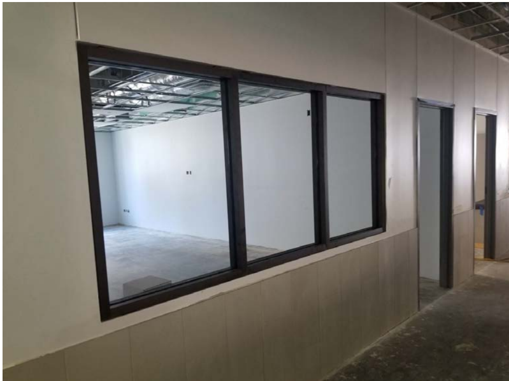
Wall Tiling and Window Frames at Classrooms
