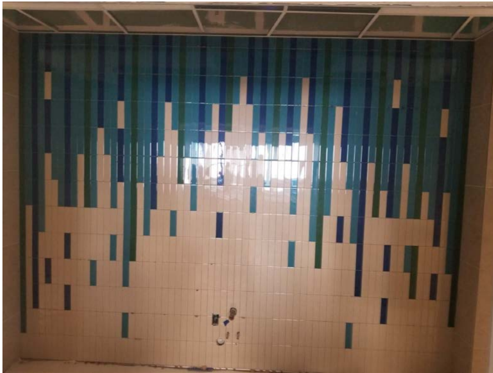
Restroom Wash Fountain Wall Tiling
