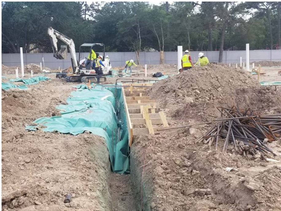
Grade Beam Forming
