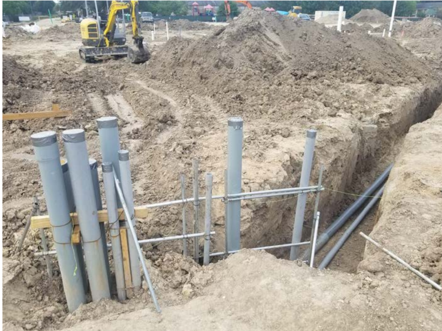
Underground utility installation
