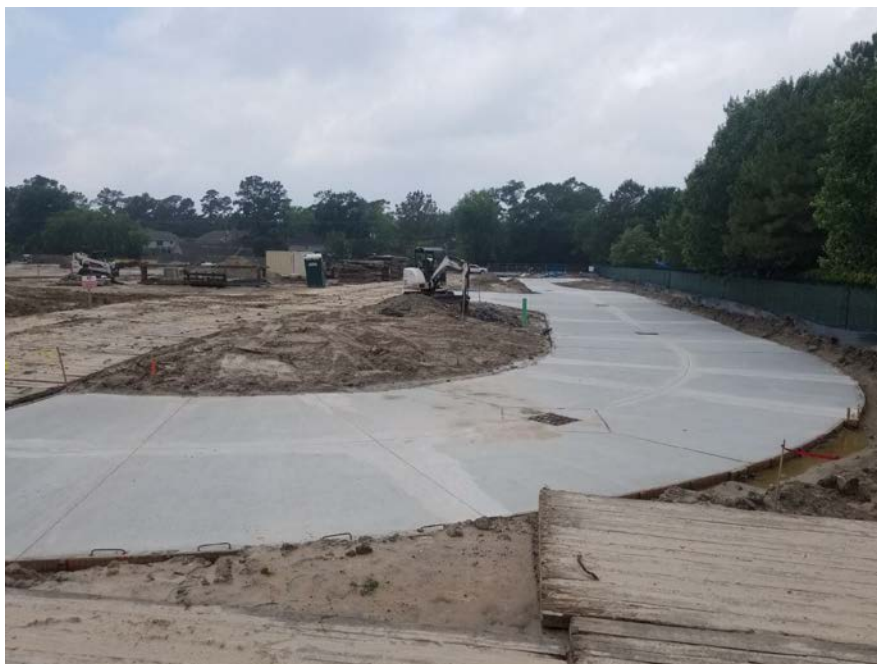
Fire Lane Paving
